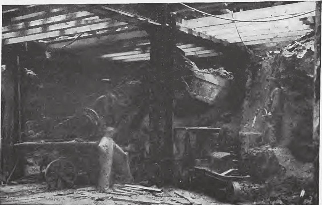
Hudson Department Store, Detroit. Making the general cellar excavation after the caissons, columns, and cellar walls had been installed in nits and the steel work erected.
