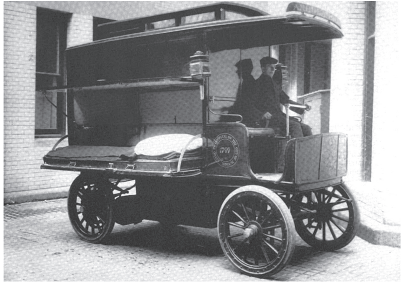
Figure 3. The Vehicle Equipment Co., based in Brooklyn, designed and produced the society's ambulance, which ran on electricity supplied by the hospital's own independent power plant. To facilitate the transfer of patients, loading occurs on the side of the ambulance. Per the Electrical World and Engineer , it could reach speeds of twenty miles per hour, and the design was so successful as to attract other buyers, including New York's Presbyterian Hospital as well as two hospitals in Paris and two hospitals in Boston. See "Hospital Electric Ambulance," Electrical World and Engineer 39, no. 18 (May 3, 1902): 783–84. Electric Ambulance of the Lying-In Hospital of the City of New York , photograph ca. 1909, National EMS Museum, Tallahassee, Florida.
