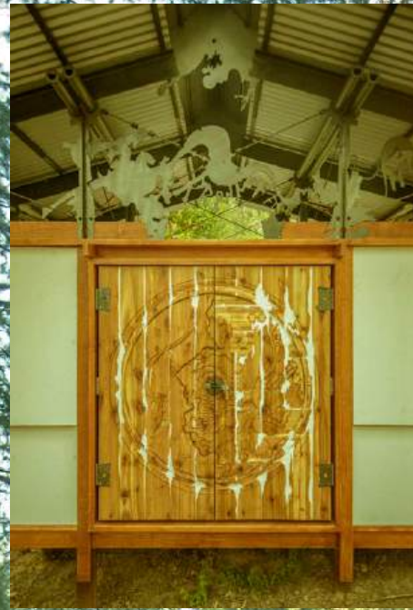
Decoration The Shinto Shed roof was made of plasma cut welded steel. The doors were made of milled cedar plank laminated together.
