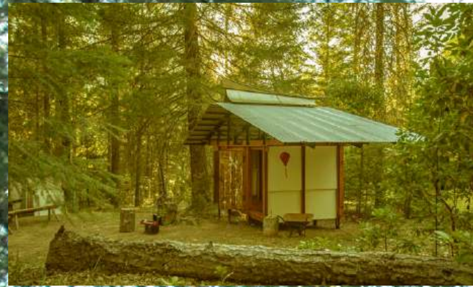
Decoration The Shinto Shed roof was made of plasma cut welded steel. The doors were made of milled cedar plank laminated together.
