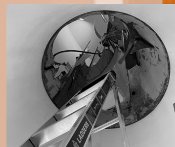
Fabrication The primary dome shell was constructed out of fiberglass leaves. The upper portion, which splinters into fragments, was made out of welded laser cut steel. The image above shows the unpainted, unbonded joint between both systems.
