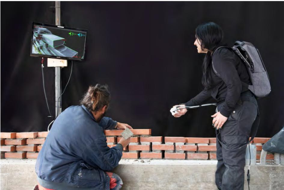
Figure 3.14: Augmented Bricklaying setup with one operator and one mason.
