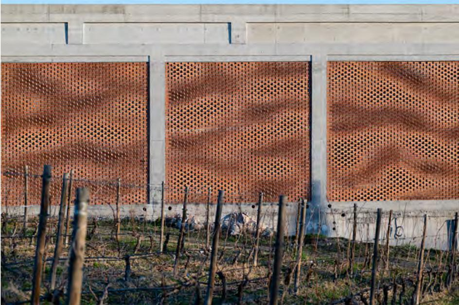
**Figure 3.12:** The design of the semi-transparent façade reflects the idea of a constantly changing pattern resembling the shimmering light of liquid
