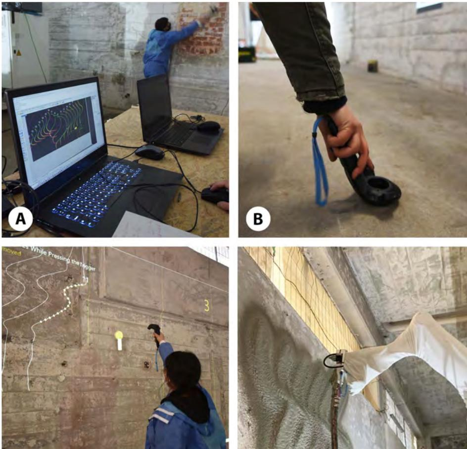
**Figure 3.21:** (A) Selection of filter (B) localisation (C) designing, adjusting the design (D) robotic spraying.
