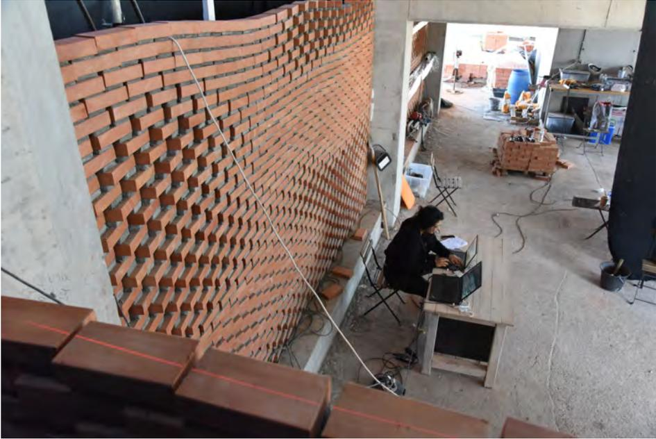
Figure 3.13: Design adjustments are made on-site to update the digital model to inform the AR interface.
