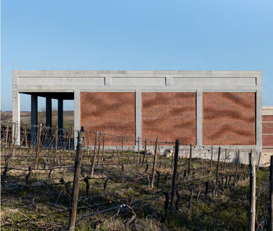
**Figure 3.2:** Katerini Winery (2019): biggest brick-structure constructed to date using augmented reality guidance
