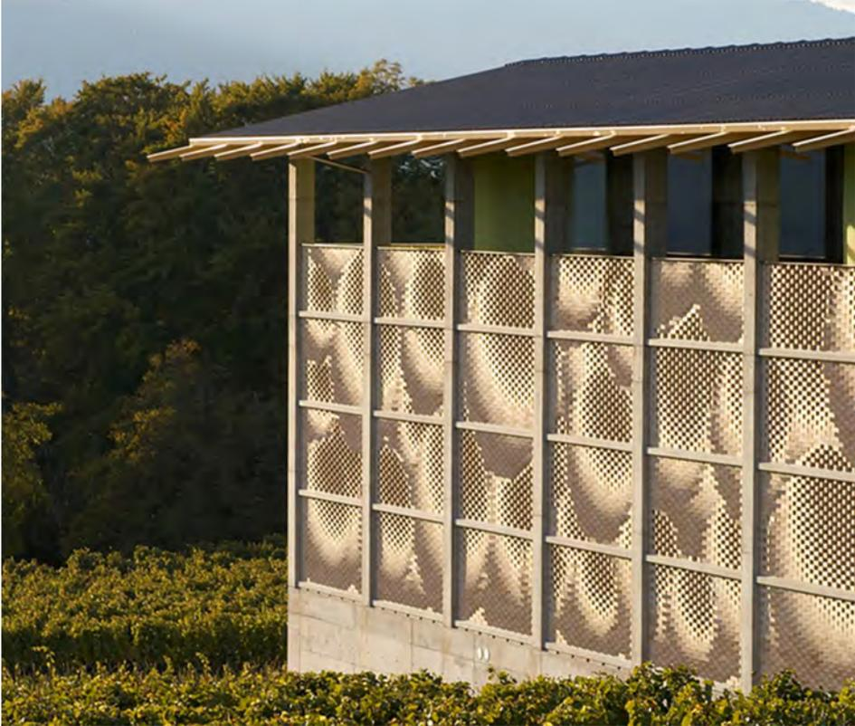
**Figure 3.3:** Gantenbein winery facade (2006): fully robotically fabricated winery
