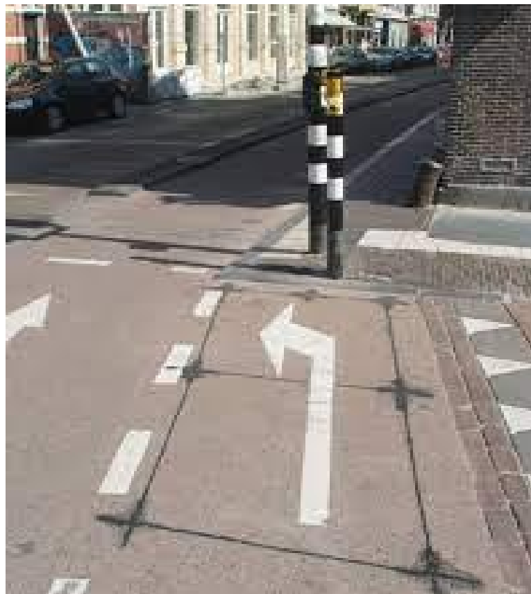
Figure 2: Loop sensors installed beneath road accompanied by ‘de knop’ at a signalized intersection
