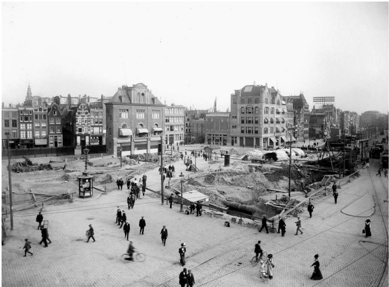
Figure 4.15: Demolition of surrounding old buildings, 1914
