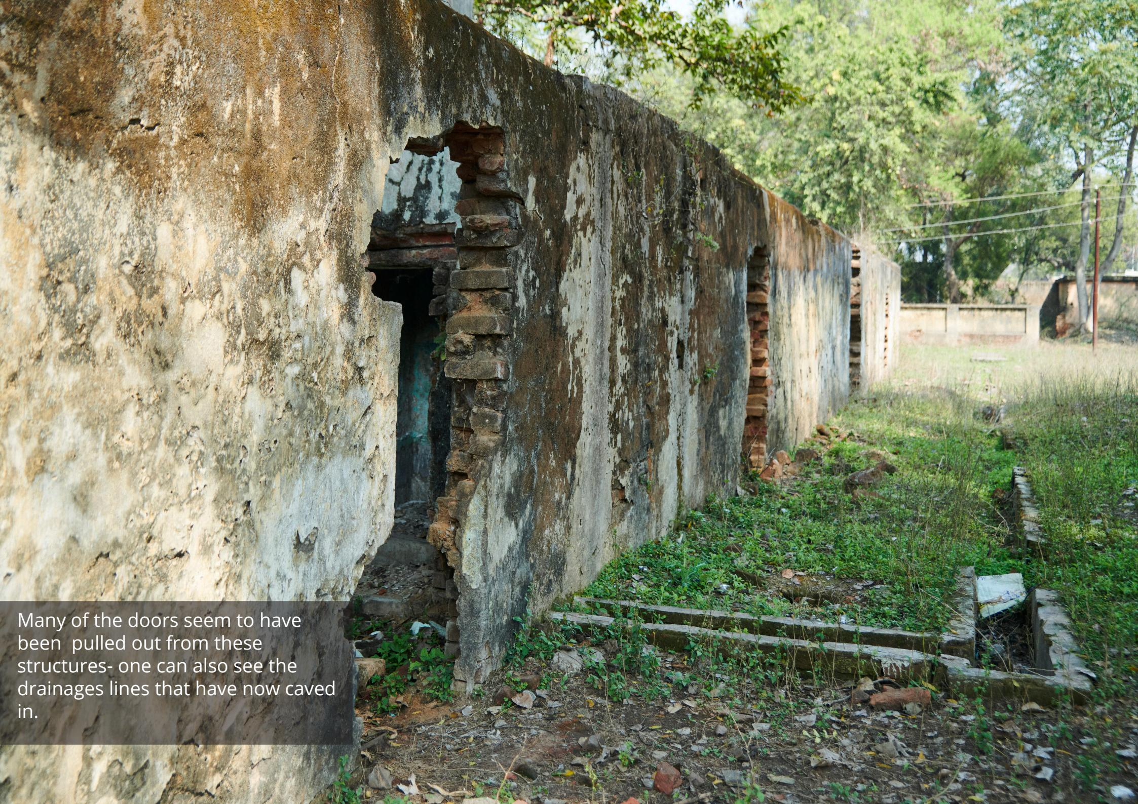
Many of the doors seem to have been pulled out from these structures- one can also see the drainages lines that have now caved in.
