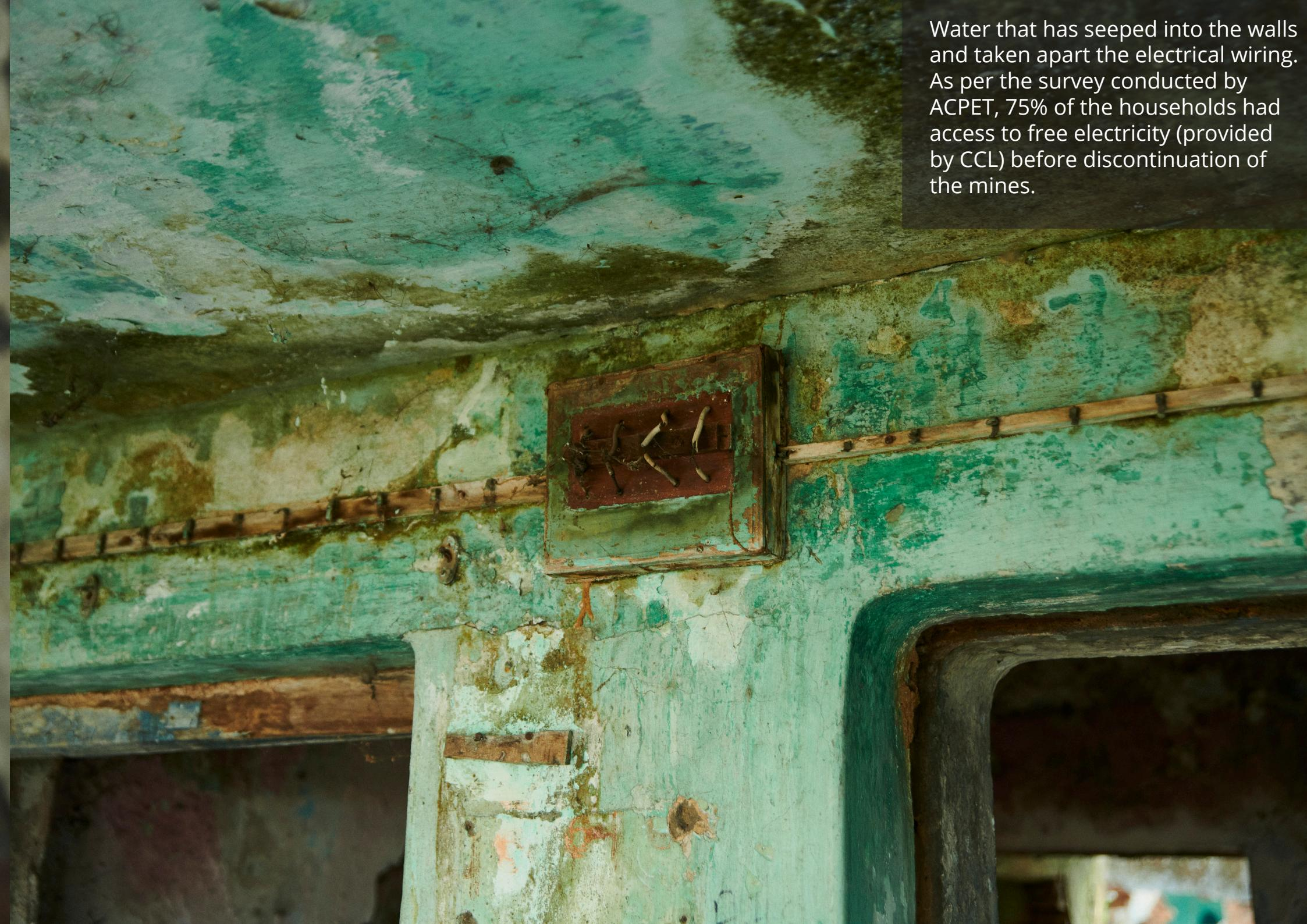
Water that has seeped into the walls and taken apart the electrical wiring. As per the survey conducted by ACPET, 75% of the households had access to free electricity (provided by CCL) before discontinuation of the mines.
