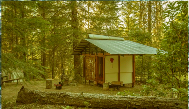
Decoration The Shinto Shed roof was made of plasma cut welded steel. The doors were made of milled cedar plank laminated together.
