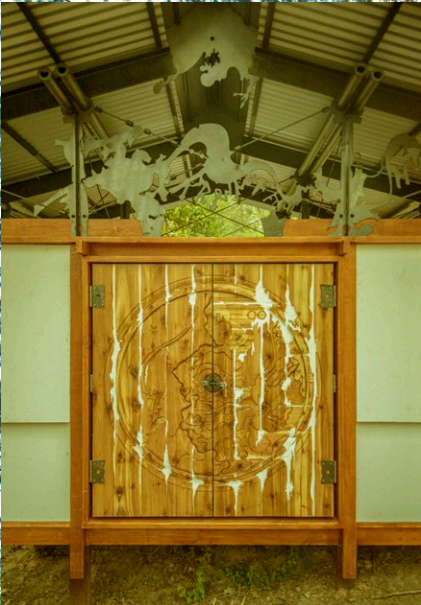
Decoration The Shinto Shed roof was made of plasma cut welded steel. The doors were made of milled cedar plank laminated together.
