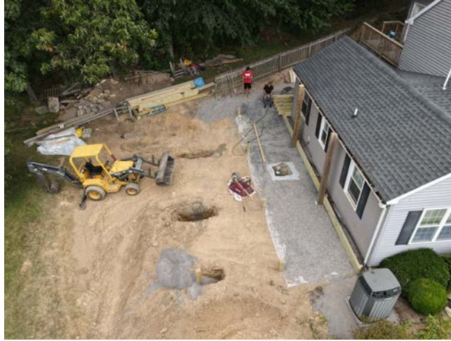
GROUND PREP AND FOOTERS
