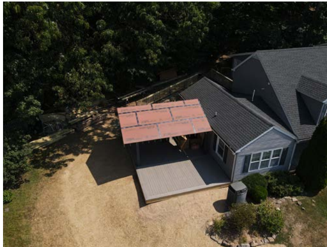
GABLE ROOF AND ZIP SHEATHING
