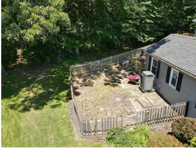
EXISTING SITE CONDITIONS
