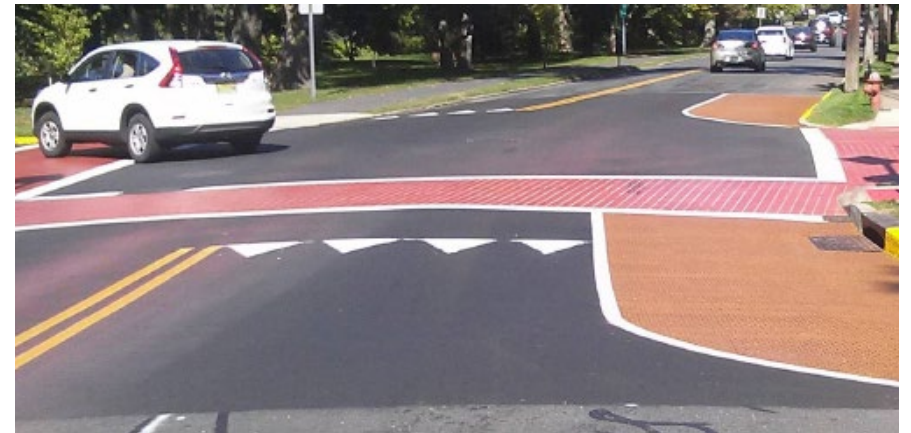
Fig. 115: Better pavement at major intersections
