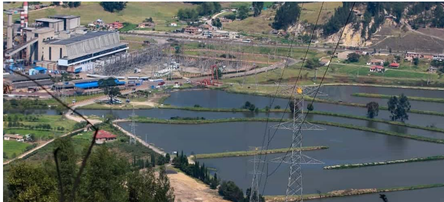
Fig. 25: Power Units around Cooling Lagoon
