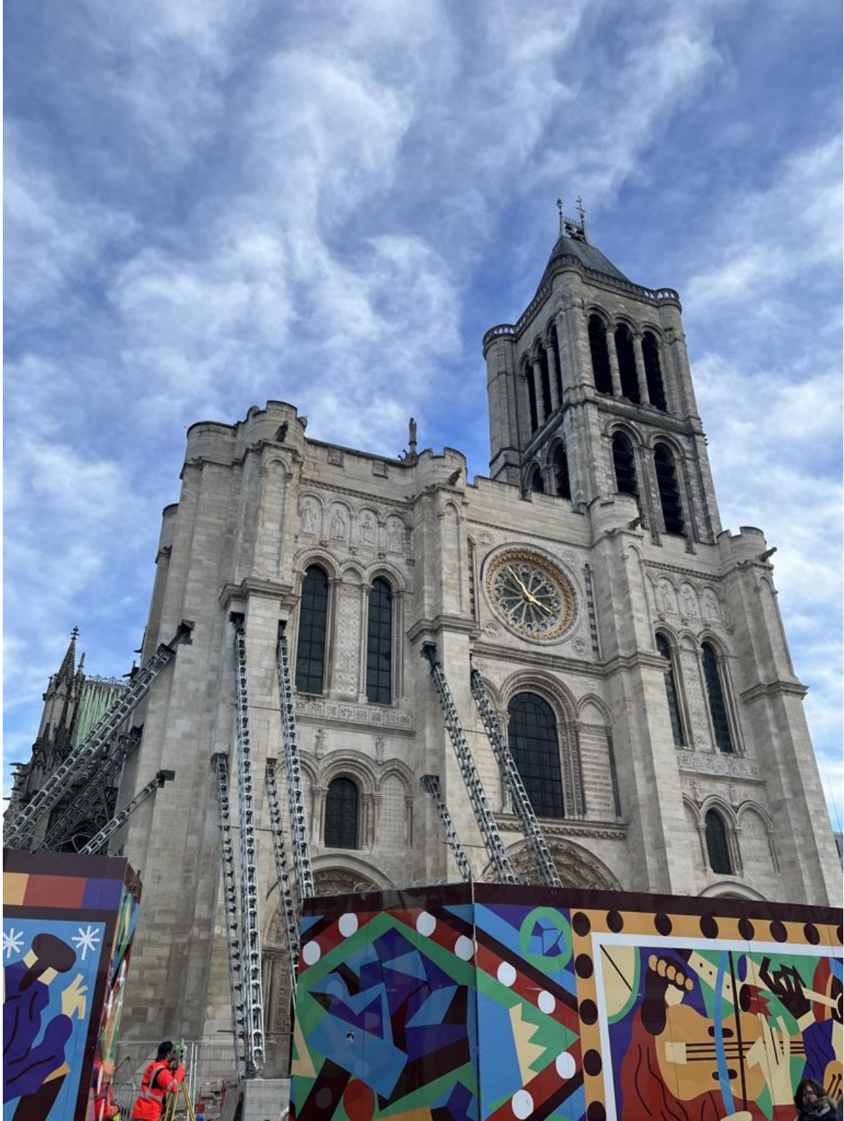
Figure 5: Construction at Saint-Denis Cathedral. Author's own, January 2023.
