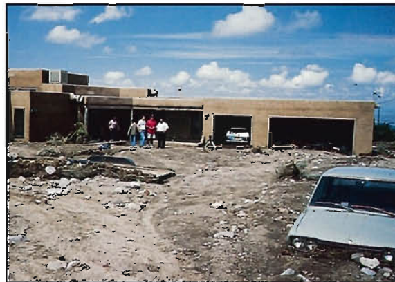
House and car damaged by floodwater and sediment, July, 1991
