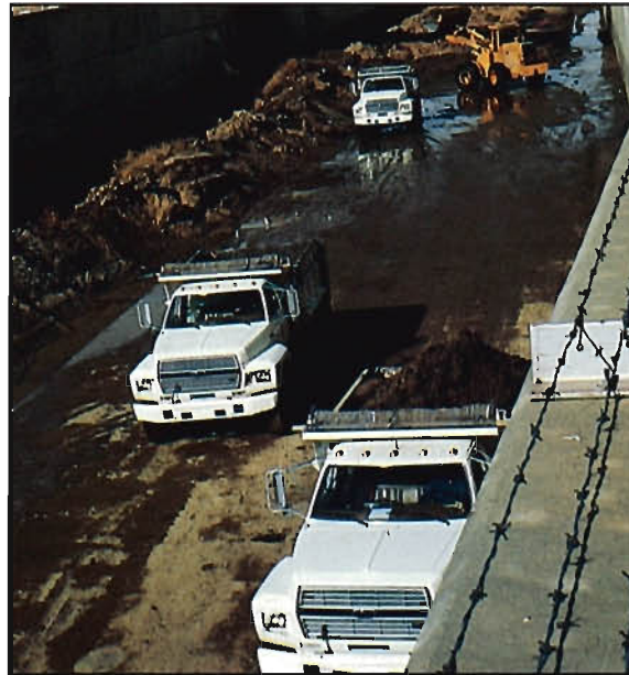
Sediment removal is a big job, averaging 80,000 cubic yards every year.
