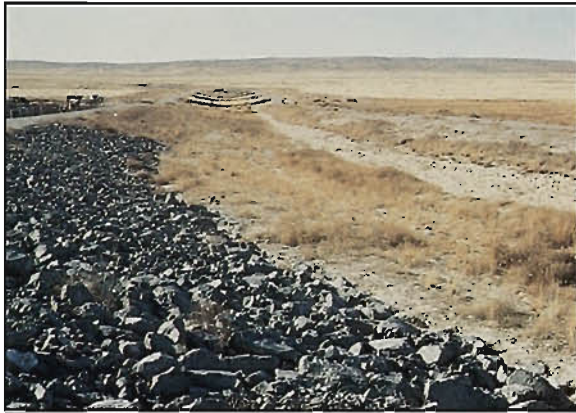
Borrega Diversion Channel, rock and grass lined
