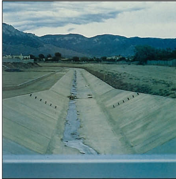
Typical AMAFCA flood control channel
