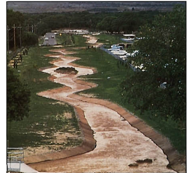
Cabezon Channel, a combination flood control and irrigation channel, in a park section.
