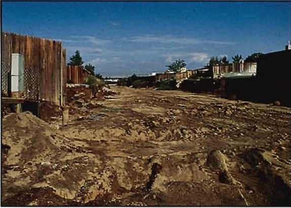
North Pino Arroyo and backyards, following 1980 storms.
