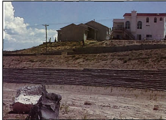
Calabacillas Arroyo soil-cement bank looks more natural than concrete
