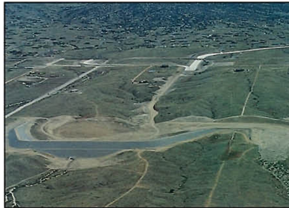
Typical AMAFCA dam
