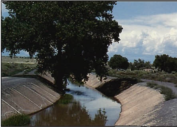
La Orilla Channel is a combination channel built with sprayed-on concrete to preserve trees and to protect a nearby archeological site.
