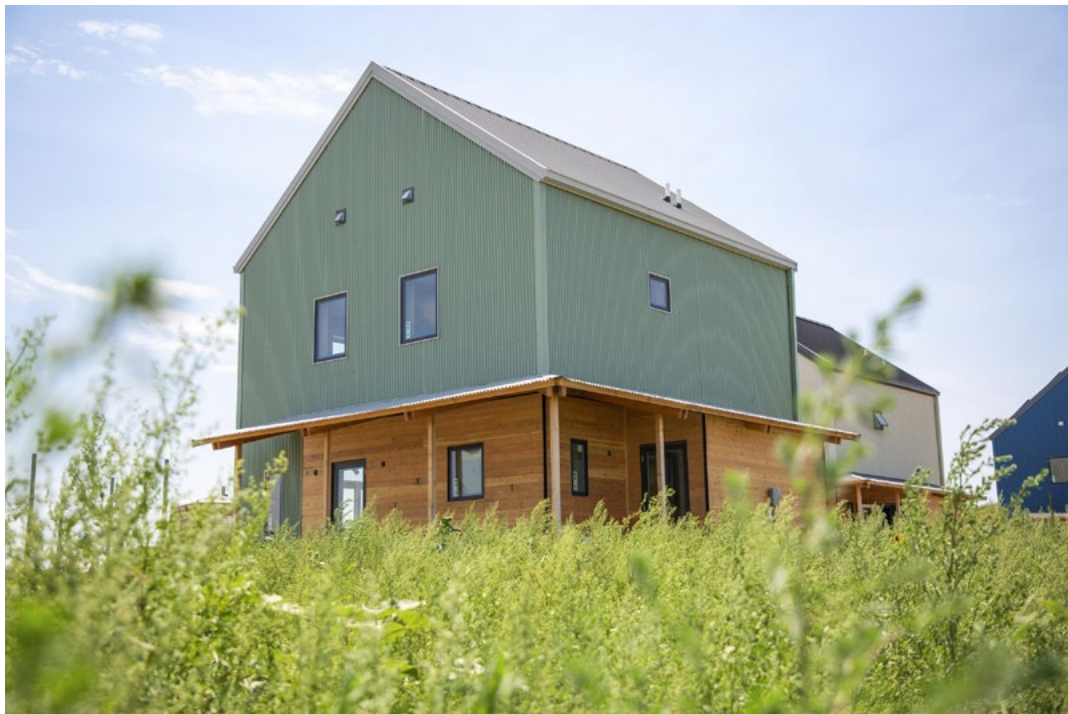
One of Thunder Valley's 21 single-family homes, each of which is equipped with east-facing entrances and solar panels.
