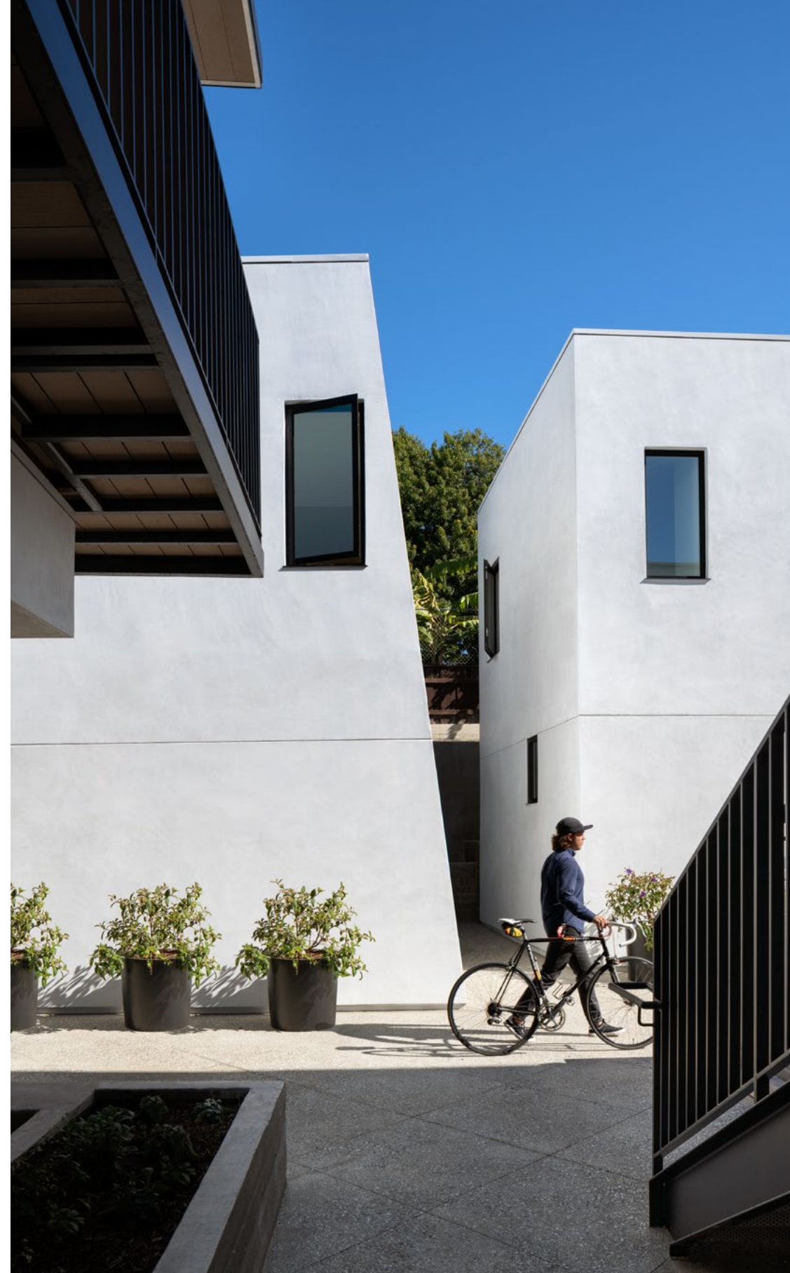
Koning Eizenberg Architecture distributed 10 units across four free-standing buildings at the Ashland Apartments, allowing patios and communal walkways to fill the spaces in between.
