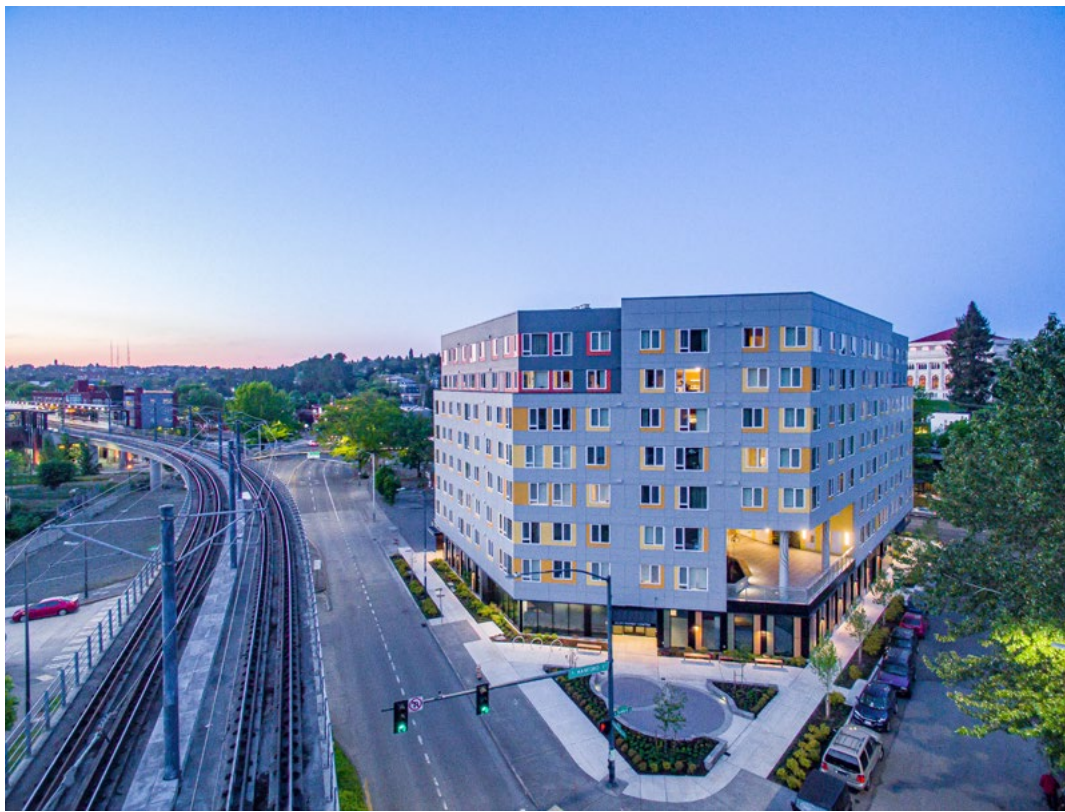
The Allen Family Center's entrance is off a mini corner plaza on the bottom floor of the Gardner House. Various building cutouts and terraces connect the building's programs to each other and to the surrounding context.
