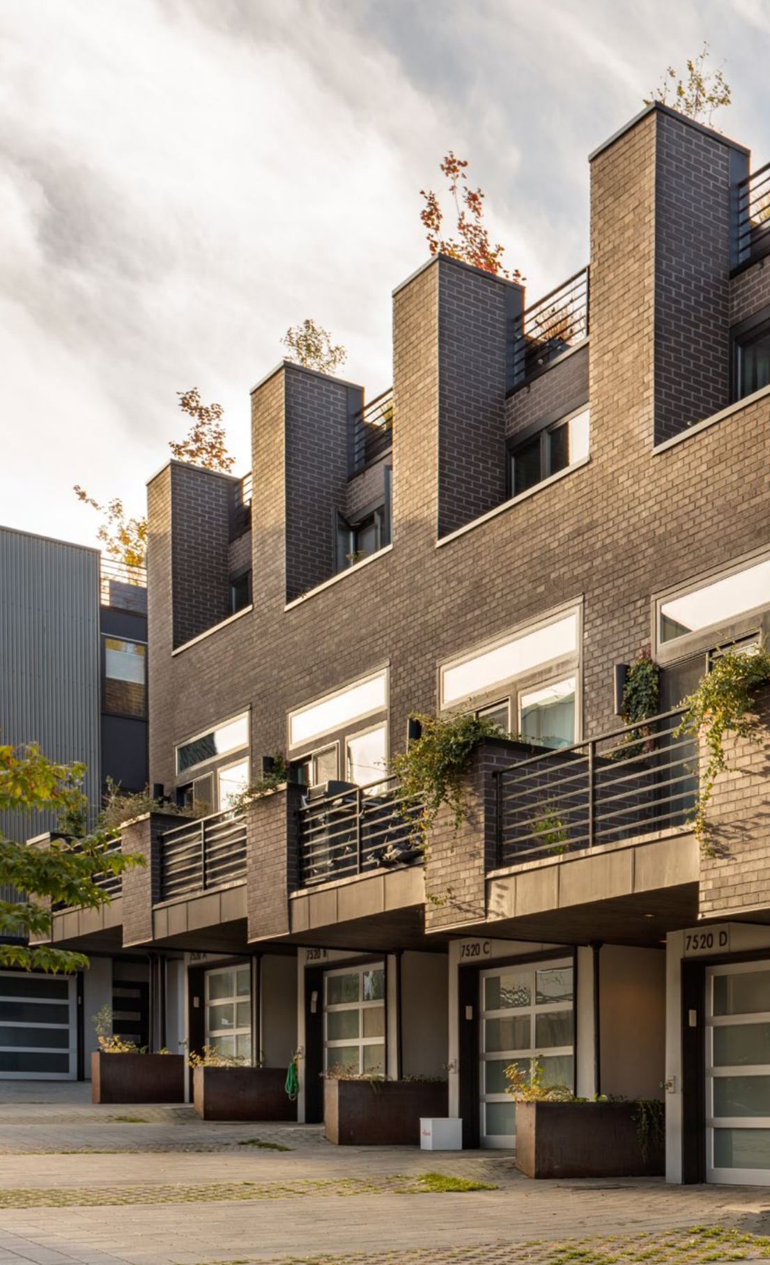
The four stories of the Othello Gardens townhomes allow for rainwater to filter at numerous points as it cascades down through a series of bio-filtration planters. PerVIOUS paving and Grasscrete contribute to water filtration.
