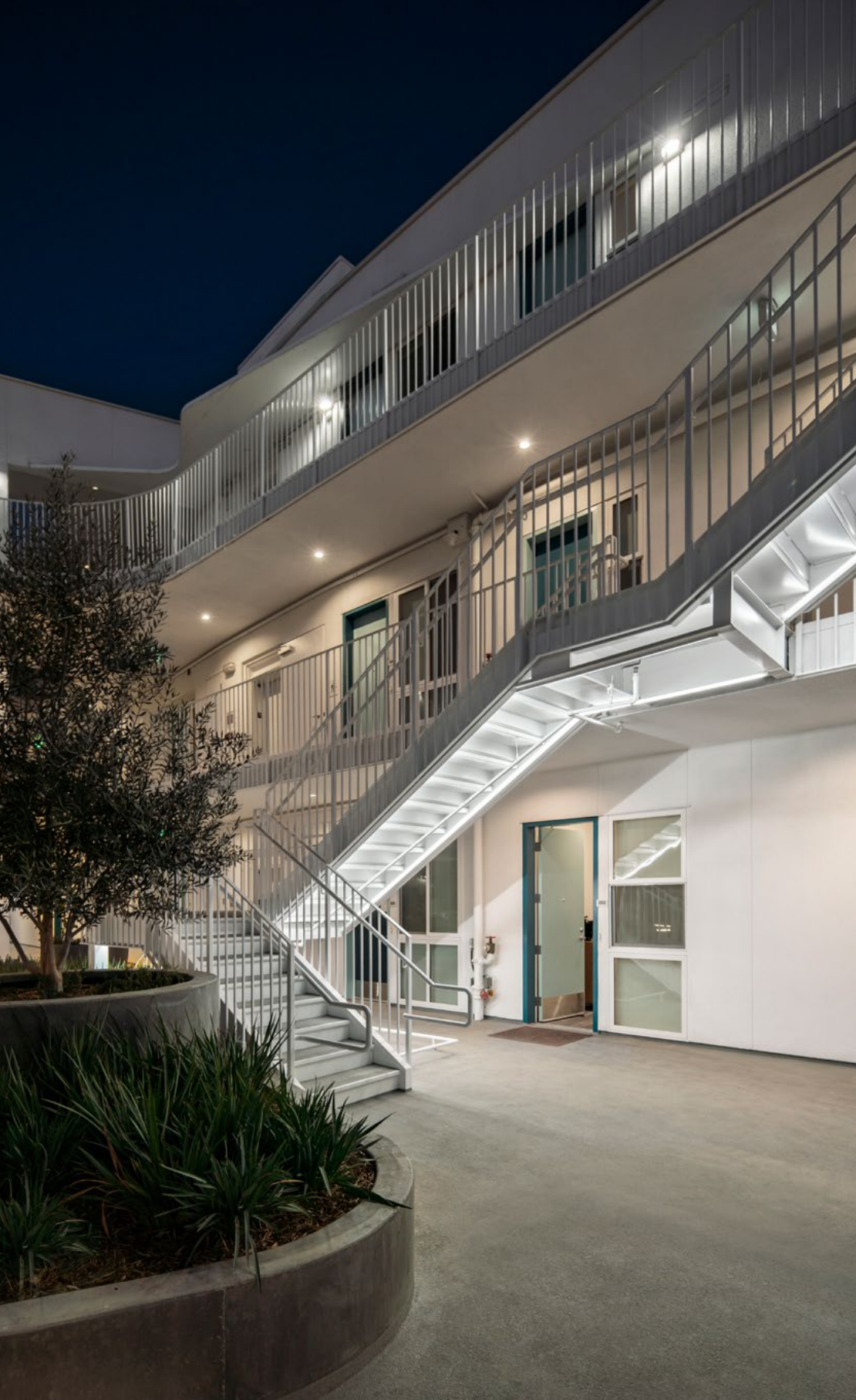
LOHA's emphasis on the single-loaded corridor opens the courtyard to residents for visual and physical interaction.
