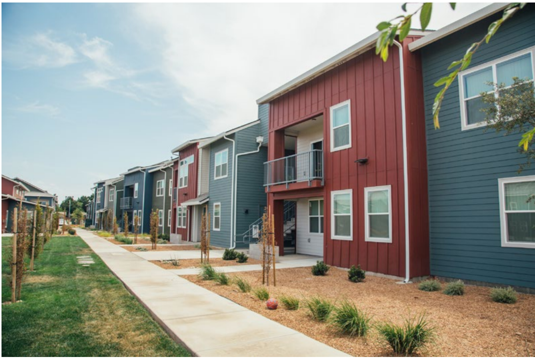
The Stonegate Village development is designed to cultivate a sense of place among residents while preventing the town of Patterson from becoming a high-cost bedroom community for the San Francisco Bay Area.
