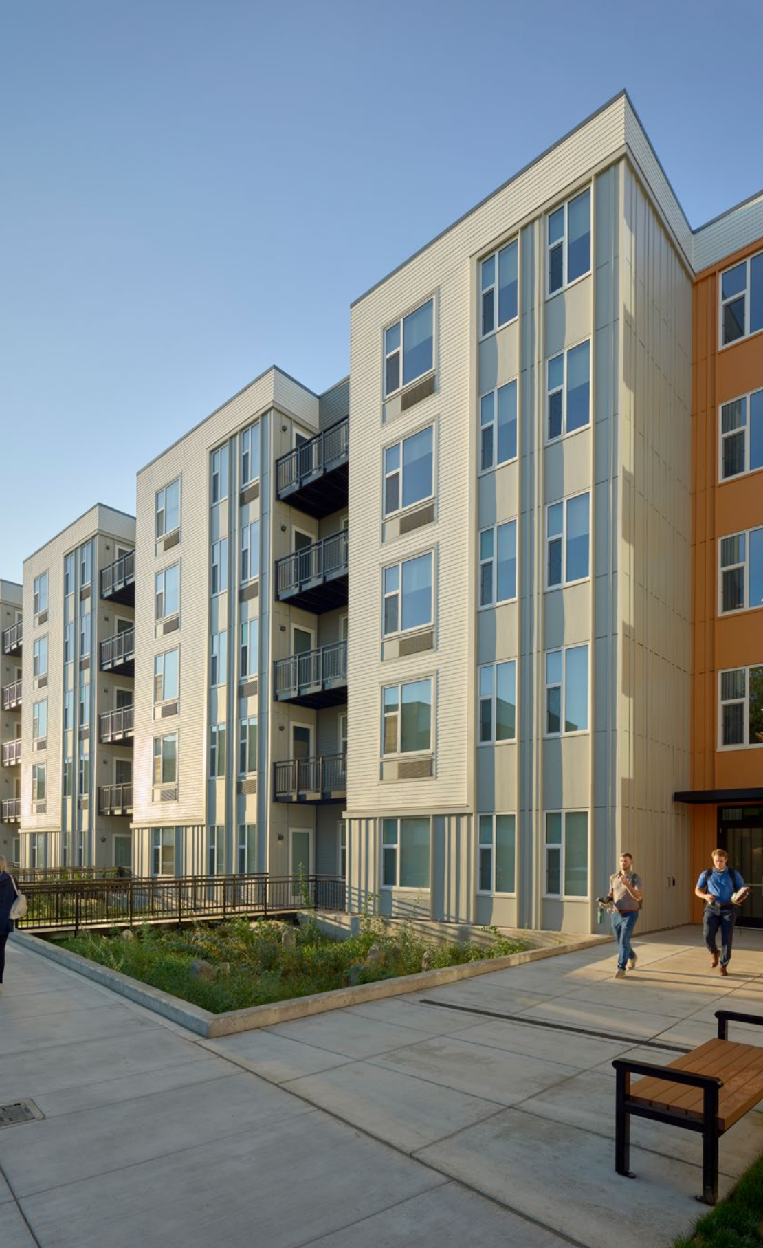
A large rain garden at Verso captures rainwater from the roof and provides a natural streetscape for residents and neighbors alike.
