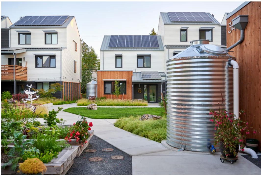
Tillamook Row's central courtyard hosts the above-ground water cistern; the project's onsite rainwater system can hold up to 3,600 gallons of water.
