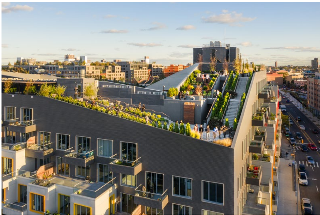
The activated roof on ODA's 10 Montieith is accessible from every residential floor and provides views over the neighborhood.
