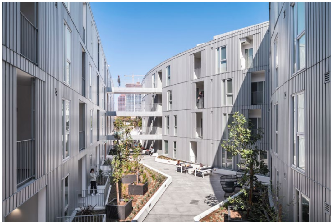
Granville 1500's curved and corrugated panels frame the buildings' courtyard.
