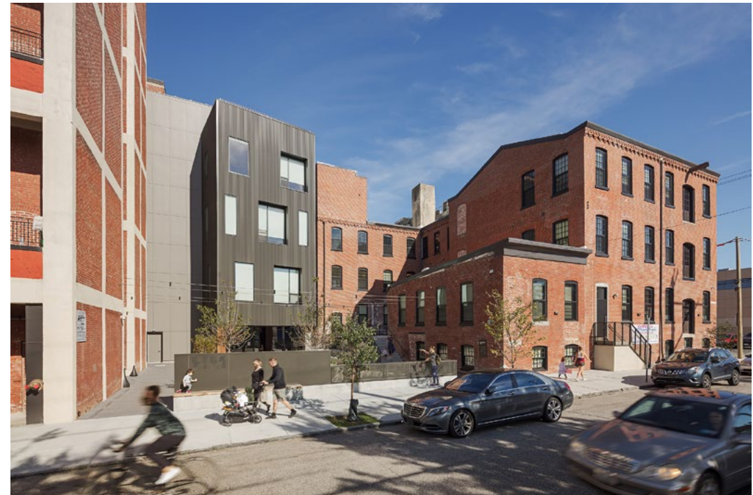
The courtyard at Huntingdon Mills both engages the street and creates a new space for gathering.
