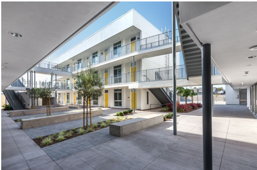
Though undetectable in its outdoor spaces, Silver Star Apartments has an onsite treatment system consisting of textile filters, microfiltration, and disinfection.
