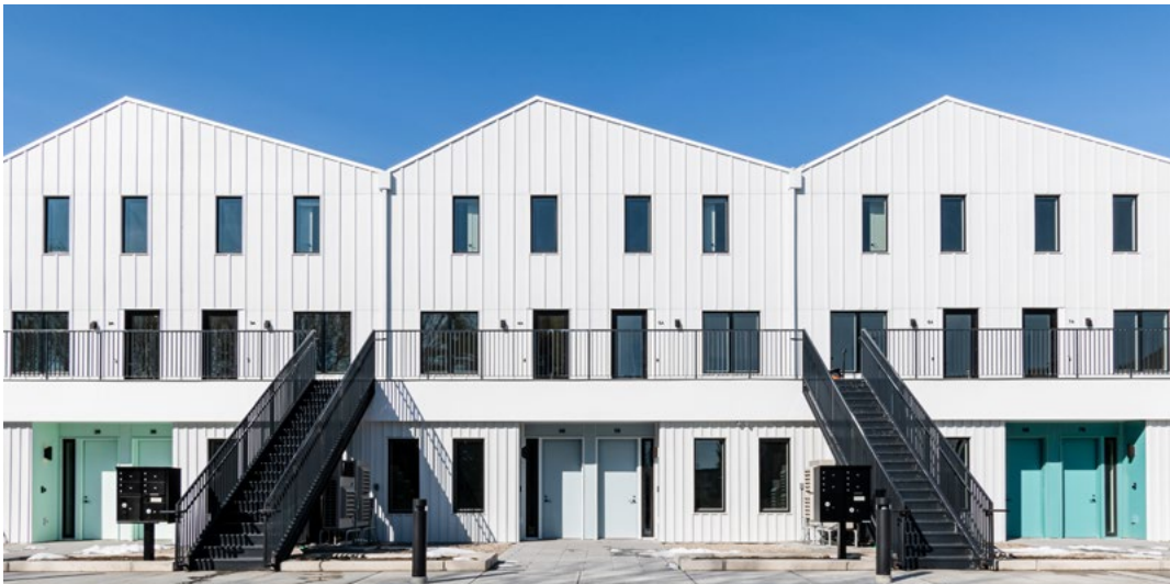
Utile's modular housing model takes on infill housing as a repeatable and scalable model for a variety of site conditions.
