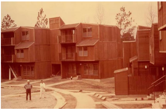
A portion of the 287 units of housing constructed in Macon, Georgia through Operation Breakthrough.
