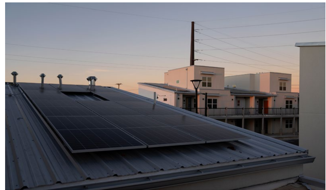
The units at Siler Yard are designed as attached townhouses with creative spaces on the ground floor.
