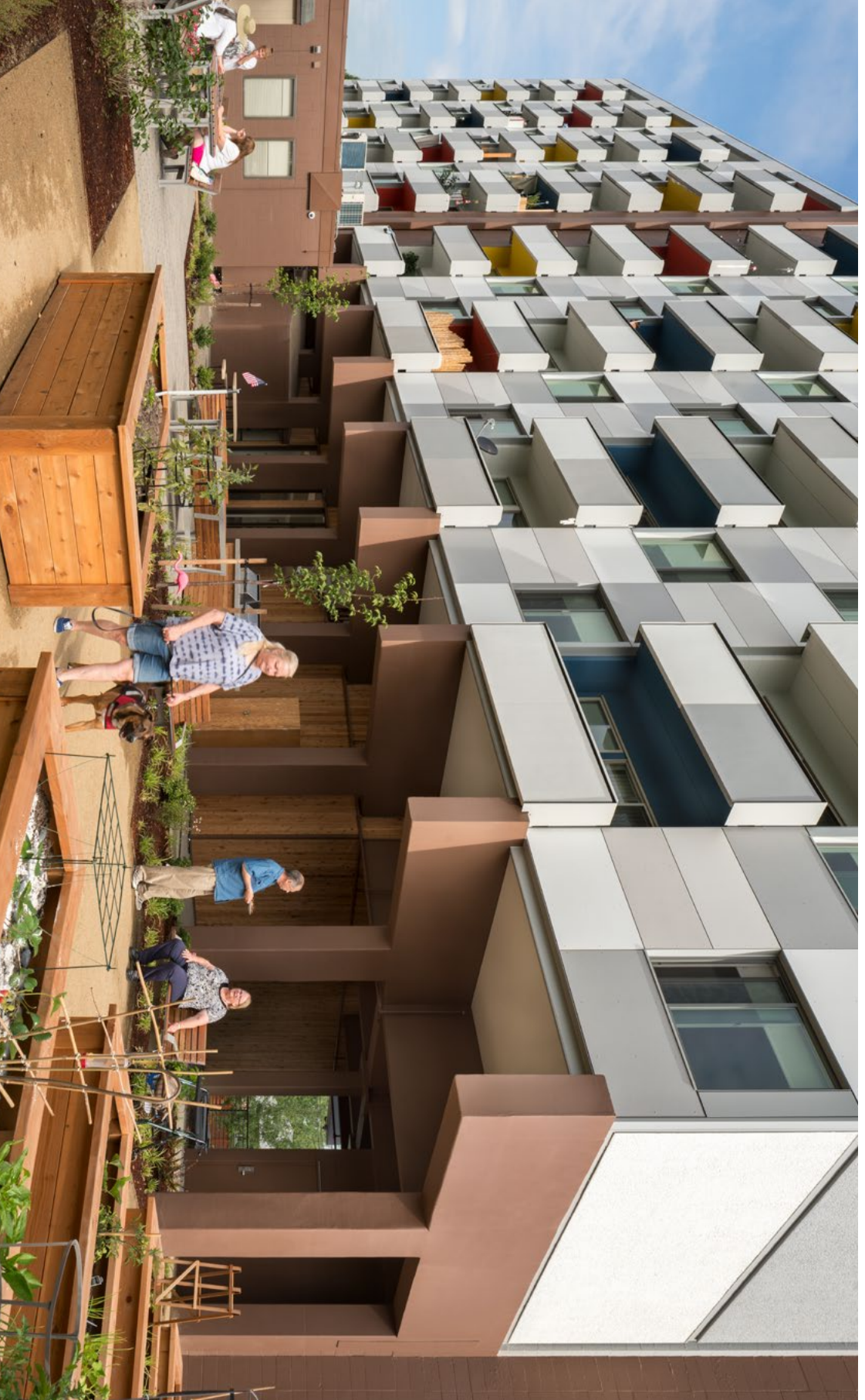
Home Forward's renovated Sellwood Center is now home to occupiable roofs with planter beds and gathering space.
