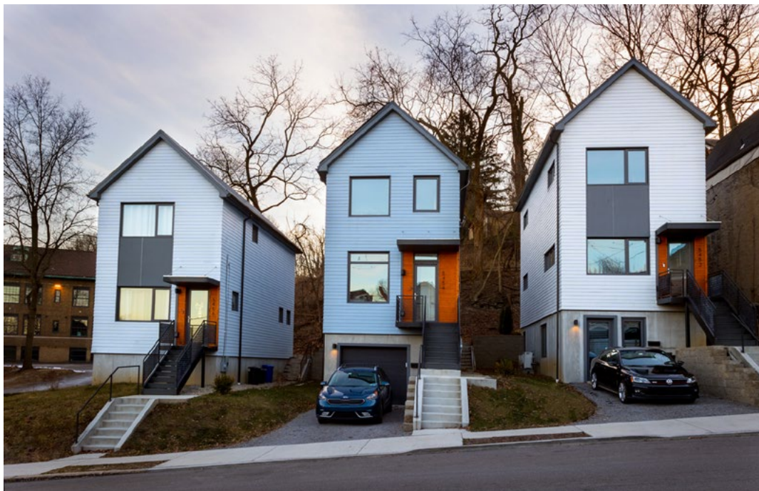
All three of the Black Street Development homes—from left; the duplex, affordable, and single-family homes—vary in square footage and bedrooms but share a material palette and street approach.
