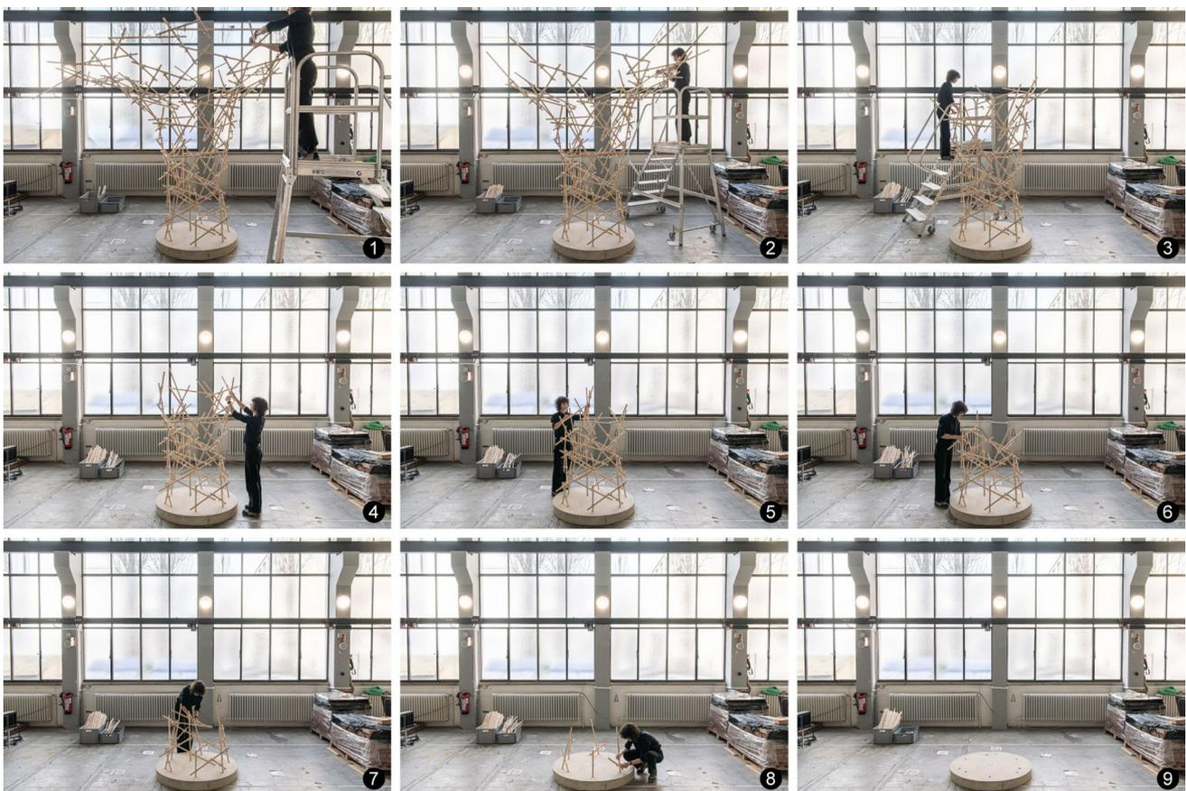
Fig. 28 Disassembly sequence in Case Study 1 showing the breakdown of the structure into its main components
