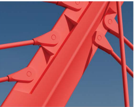
Steel Columns Galvanized steel framed column with a red powder coating. Flat finish with and alkyd primer. Paint the location of the lap joint after welding.
