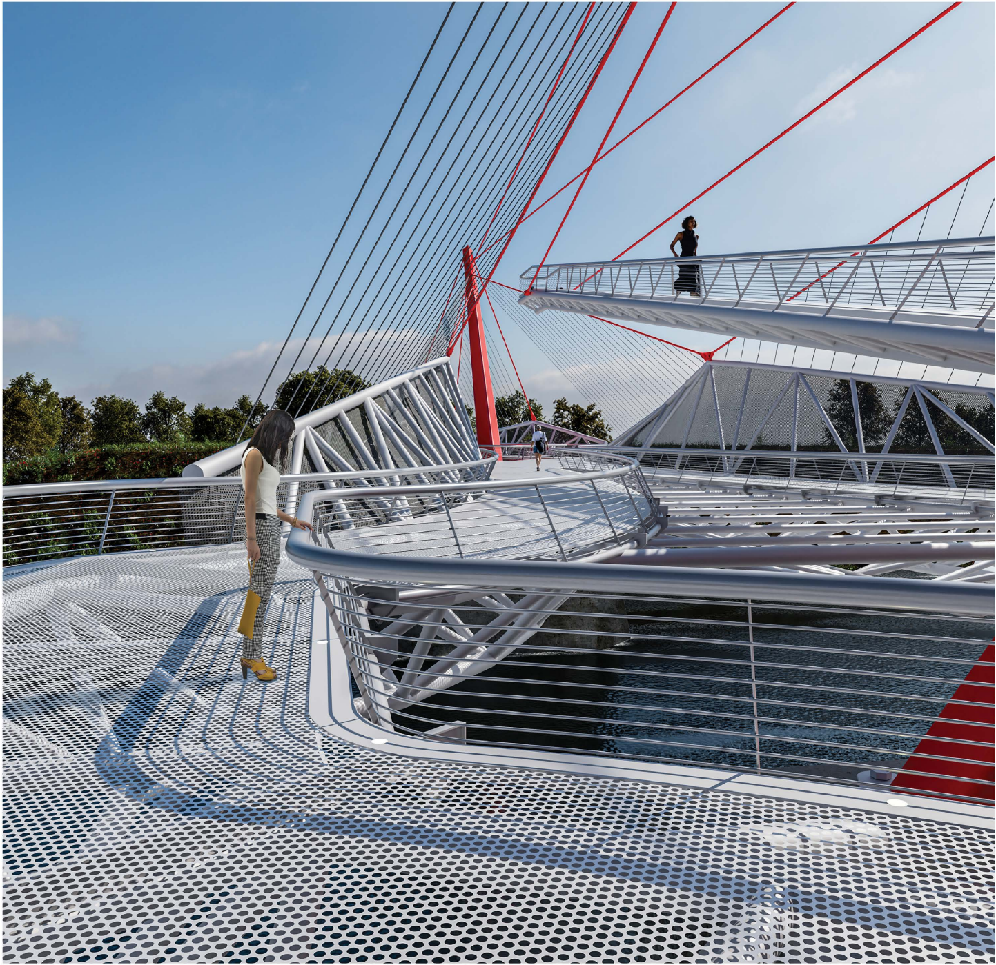
Steel Columns Galvanized steel framed column with a red powder coating. Flat finish with and alkyd primer. Paint the location of the lap joint after welding.
