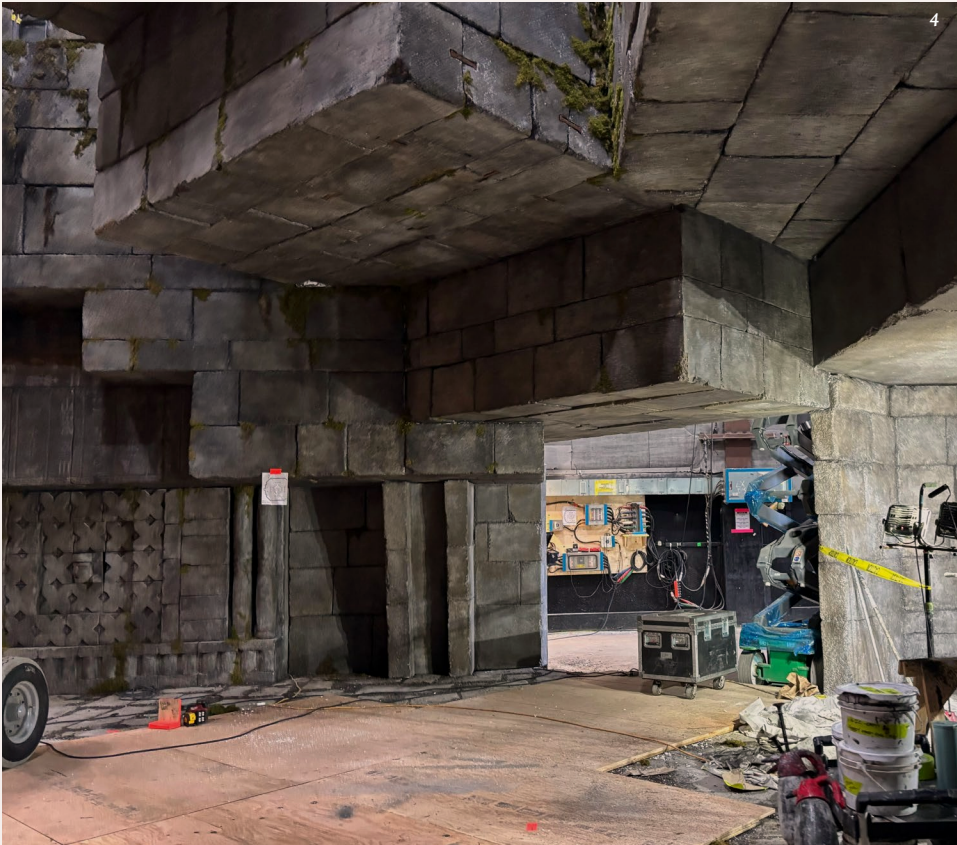
3 Foam core massing model used for rigging mock-up and proportion study 4 The suspended modules meeting the perimeter stop 5 Steel frame hold ply and coated styrofoam 6 Installation of ceiling grid and modules on stage
