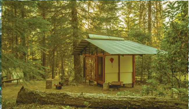
Decoratio The Shinto Shed roof was made of plasma cut welded steel. The doors were made of milled cedar plank laminated together.
