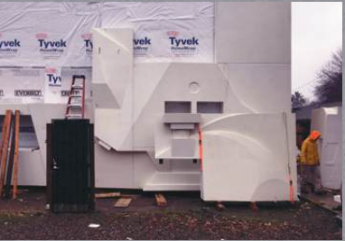
D-FAB One fabrication drawing, and one CAM file produced all constitutive components for the creation of the facade.
