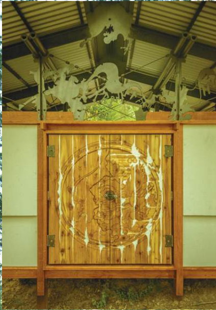
Decoratio The Shinto Shed roof was made of plasma cut welded steel. The doors were made of milled cedar plank laminated together.
