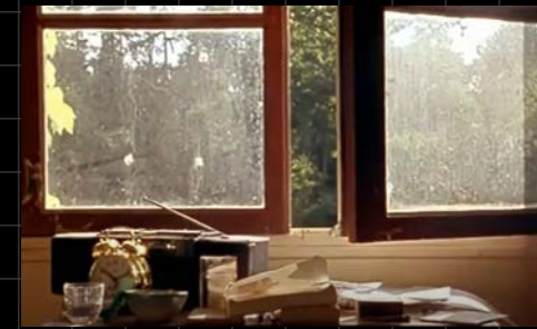
interior gives no sense of institutionalization with operable windows and open door policies
