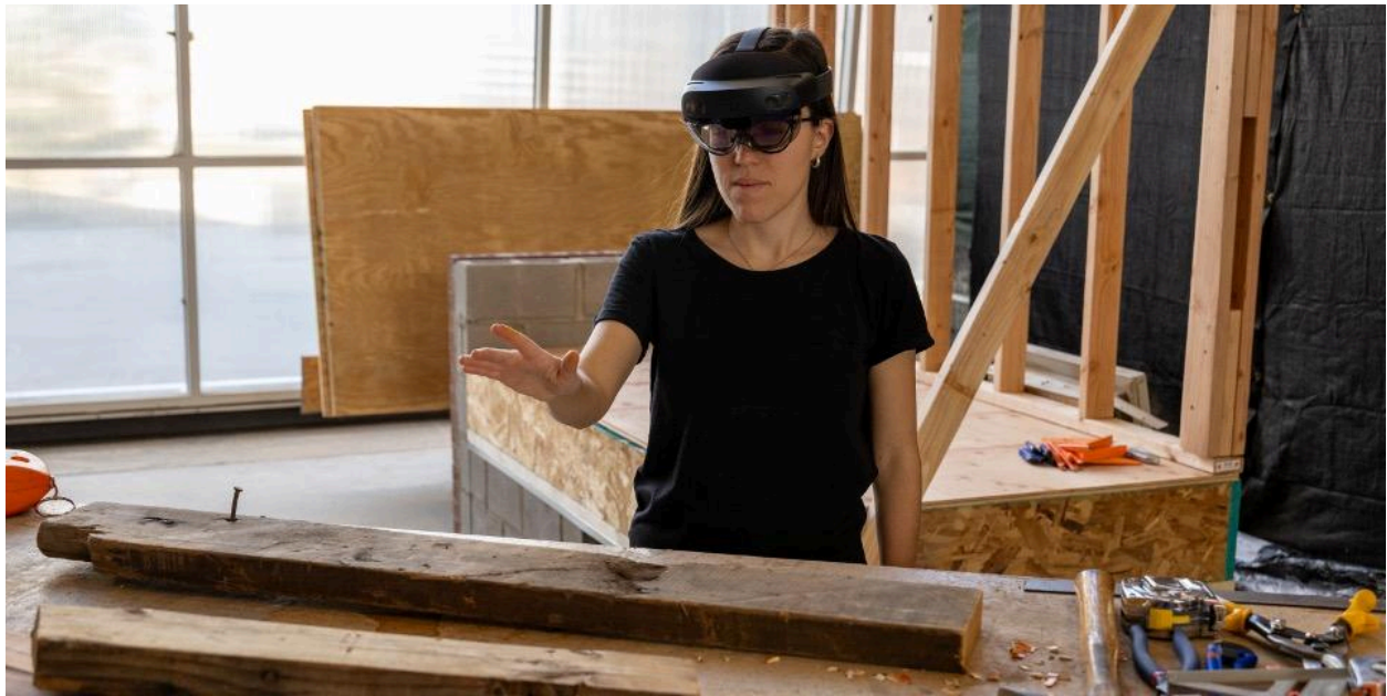
Fig.3: A worker wears an AR headset to follow real-time assembly instructions for placing irregular wooden shingles, guided by a shared digital model on-site.
