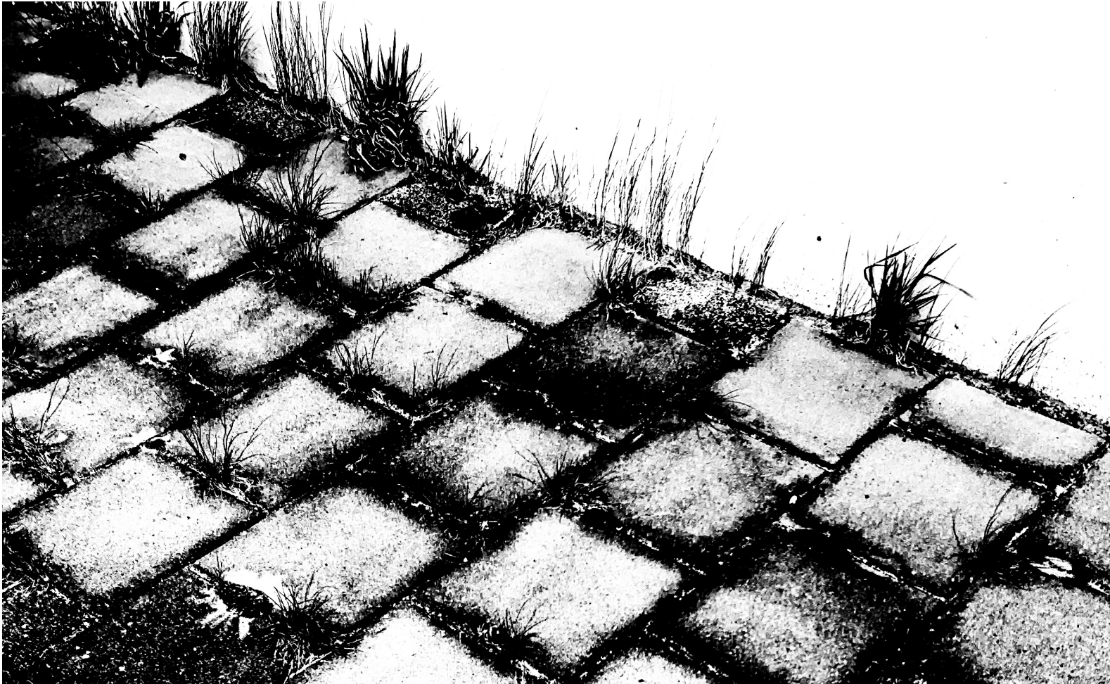
Figure 22: Captured in Rotterdam Noord, 2024. Tiles with grass growing between the cracks.
