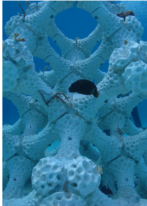
Figure 57: MODULAR ARTIFICIAL REEF STRUCTURE made of 3D printed ceramics. Image from Reef Design Lab (2018)
