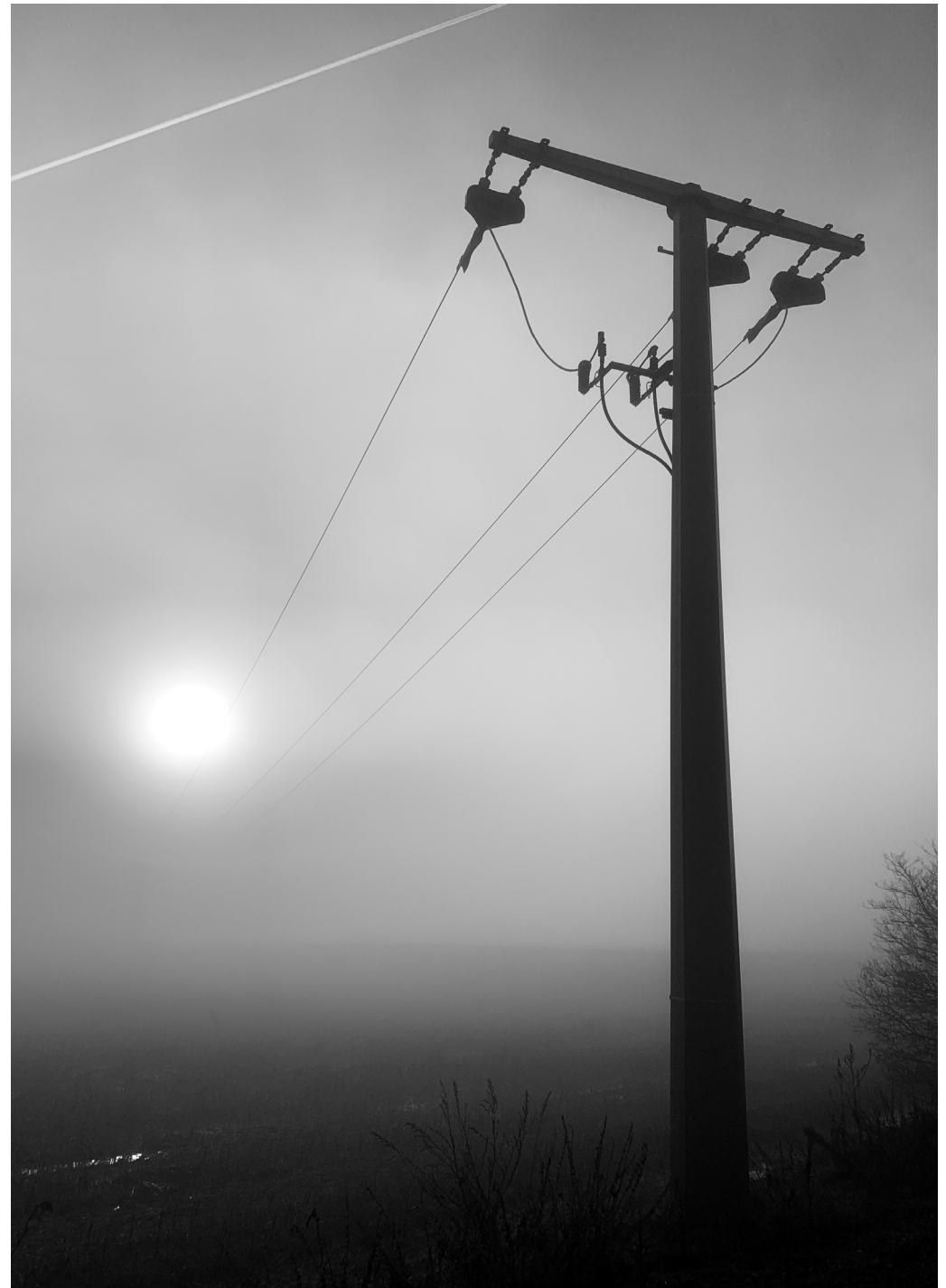
Figure 60: Image captured in Germany. Power pole in a field with airplane contrail in the sky.
