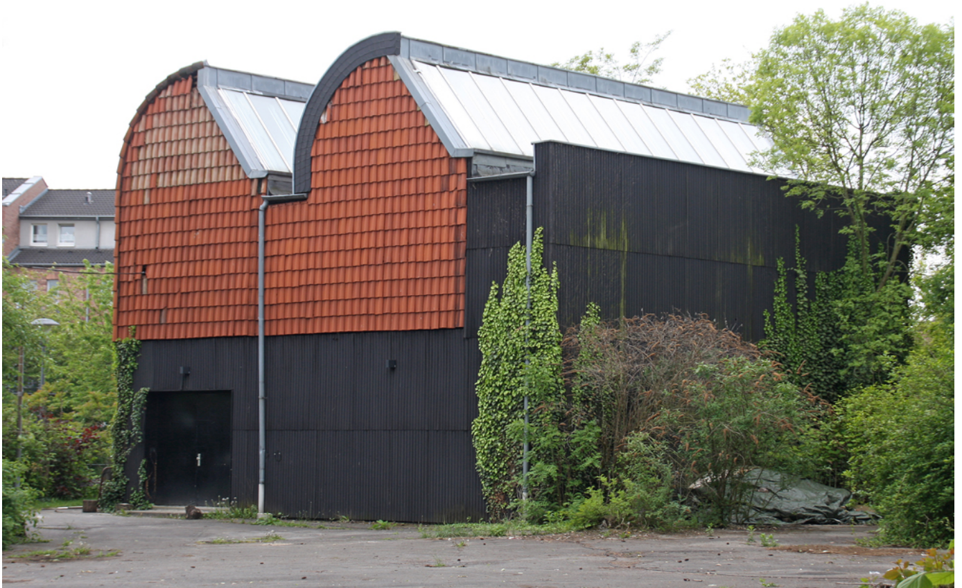
Simultanhalle was built in 1979 as a model for the planned Museum Ludwig by the architects Busman+Haberer to test mainly the lighting of the space through the characteristic shed roof construction. Since 1983, it has been used as project space for contemporary art in Cologne.
