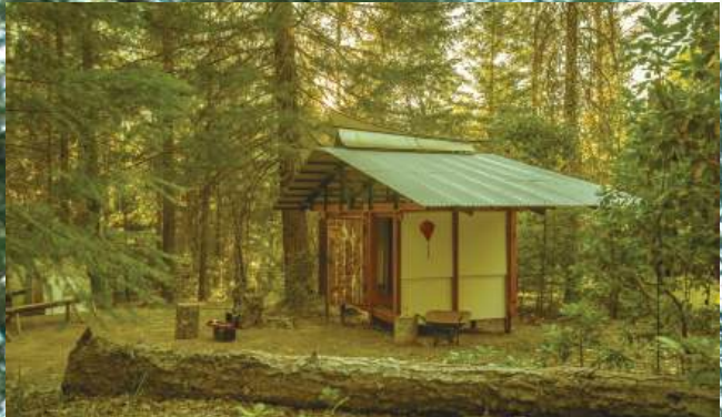
Decorative The Shinto Shed roof was made of plasma cut welded steel. The doors were made of milled cedar plank laminated together.
