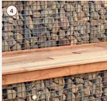
Buff reclaimed sandstone gabion walls to perimeter plinth of building
