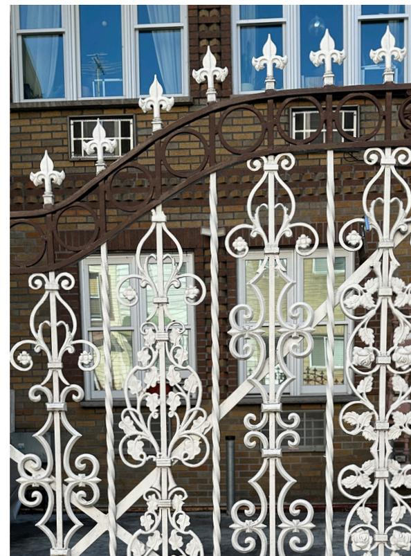
Fig. 19. Cast iron fence (potentially with some wrought iron elements) in Greenpoint, Brooklyn. Photograph by Abby Lee, 2024
