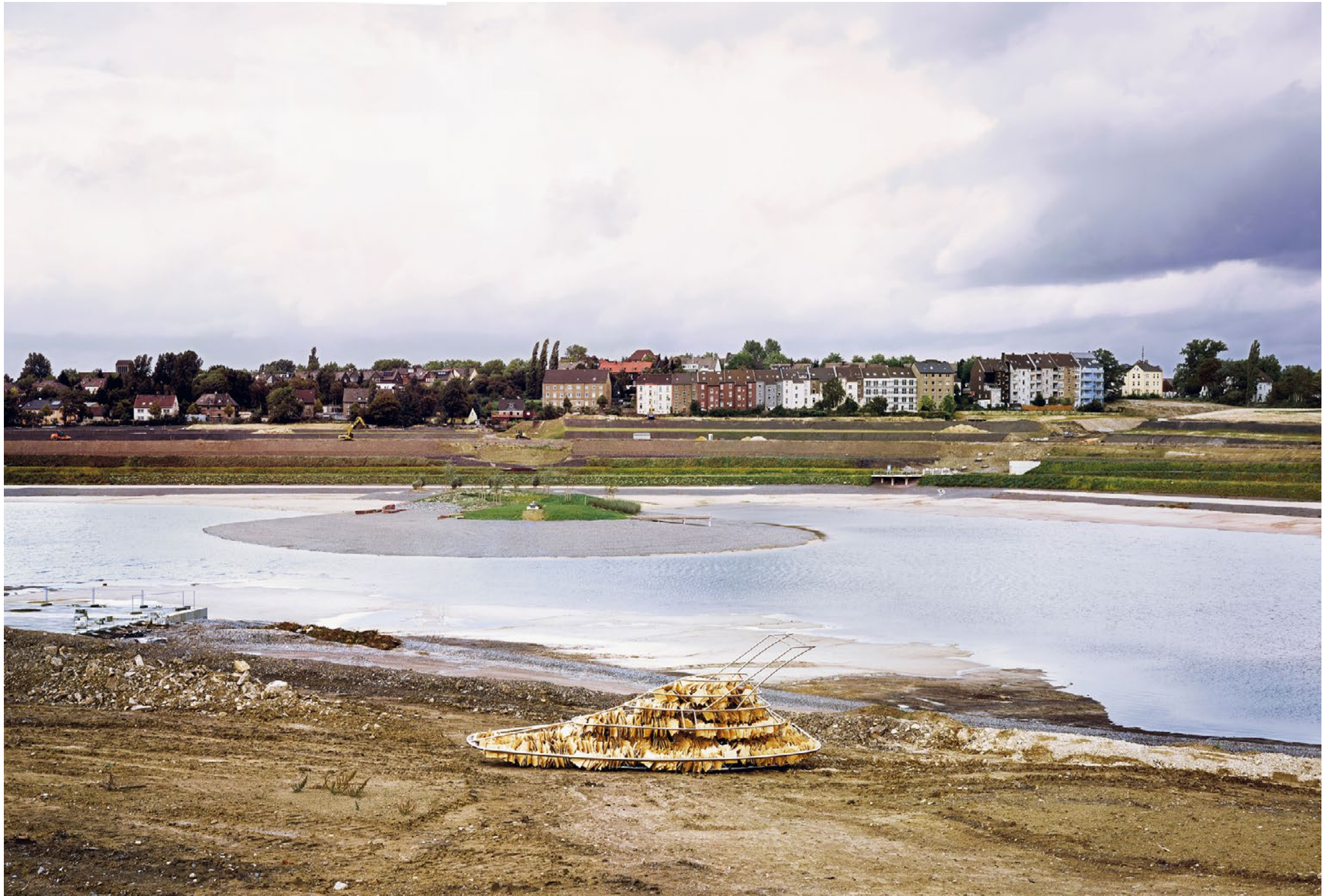
Site Photography - Temporary Harbour at LAKE PHOENIX 2010
