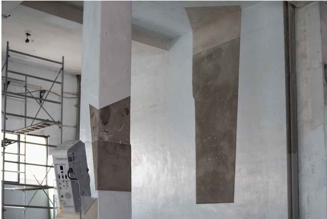
Infra- Image (N25°3'50.18", E121°25'58.33 ")", 2022 | After wall sanding
