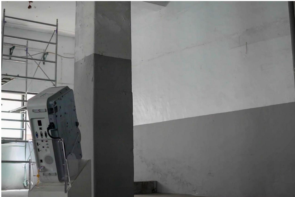
Infra- Image (N25°3'50.18", E121°25'58.33 ")", 2022 | Before wall sanding
