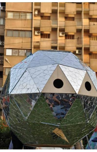
The sphere was built as two geodesic domes that fit perfectly onto each other and these domes were further broken into 2 types of triangles that were attached together by joints that could be connected and disconnected. The idea was to construct something that can be assembled and disassembled easily on-site and then stored in a compact form in Mahatat's office for future use.
