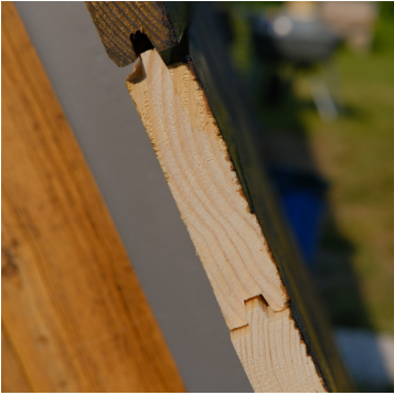
Oops! One of our mistakes: Wood paneling was installed with different sides up — notice the opposite wood grain direction
