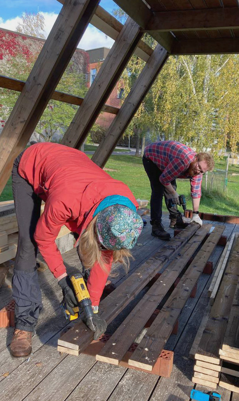
Mission 1: Installing the final layer of charred wood
