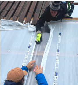
Mission 2: Installing polycarbonate sheets (and discovering new tools: credit cards for slotting the sheets together)
