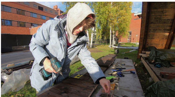
The roof was made of leftover charred wood (featuring Em, the on-site queen)
