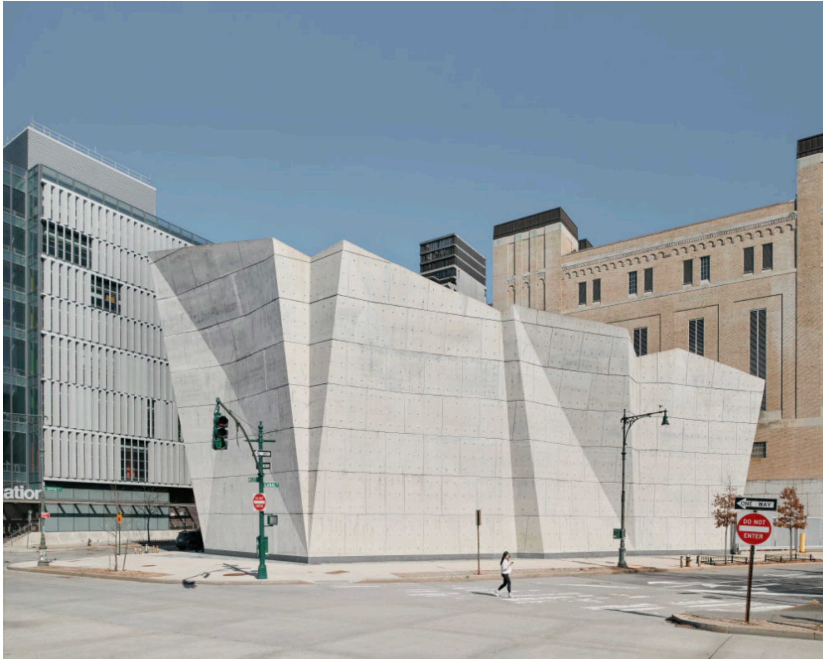
Spring Street Salt Shed NEW YORK, NY / Dattner Architects
