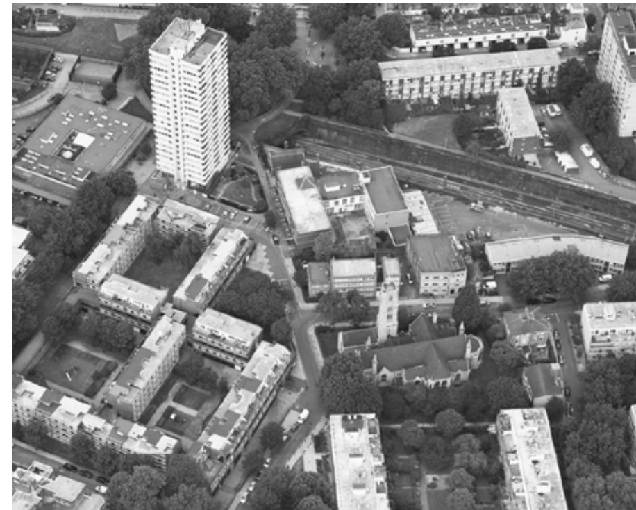
An aerial view of the Bacton Estate, before demolition. (Photo: Karakusevic Carson Architects)
