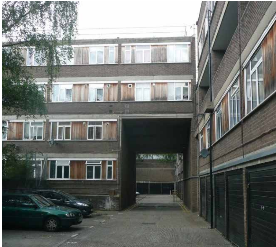
An interior courtyard on the original Bacton Estate (Photo: Karakusevic Carson Architects)
