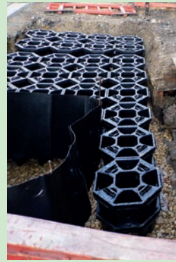
Installation on Richmond Hill, Bournemouth
