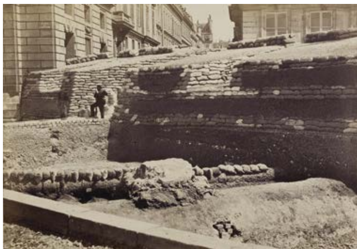
↑ Paris Commune barricade at Place de la Concorde, 1871. Shoemaker Napoléon Gaillard showed a talent for such constructions and designed them. Photo by Augustin-Hippolyte Collard.
