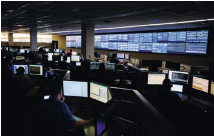
↑ Blackberry network operation center, Waterloo, Canada. ← CERN Computer Center, Meyrin, Switzerland, 2014.
