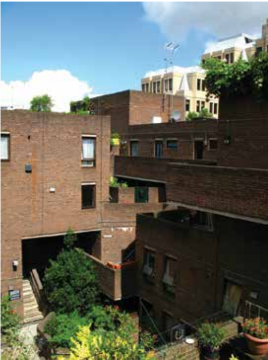
The structure of Odham's walk is based on a concrete frame with hollowcore floor slabs. This system is then covered in a multi-colored stock brick to seamlessly fit the complex into the surrounding Covent Garden neighborhood. Looking closely, however, much of the concrete structure is still visible. The roof insulation is provided by an "inverted roof." The dwellings are heated by individual and centralized gas-fired boilers with central metering.
