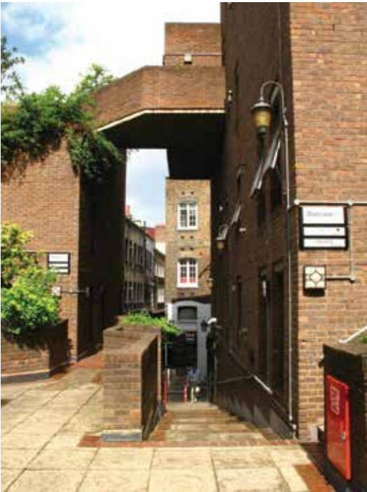
The structure of Odham's walk is based on a concrete frame with hollowcore floor slabs. This system is then covered in a multi-colored stock brick to seamlessly fit the complex into the surrounding Covent Garden neighborhood. Looking closely, however, much of the concrete structure is still visible. The roof insulation is provided by an "inverted roof." The dwellings are heated by individual and centralized gas-fired boilers with central metering.
