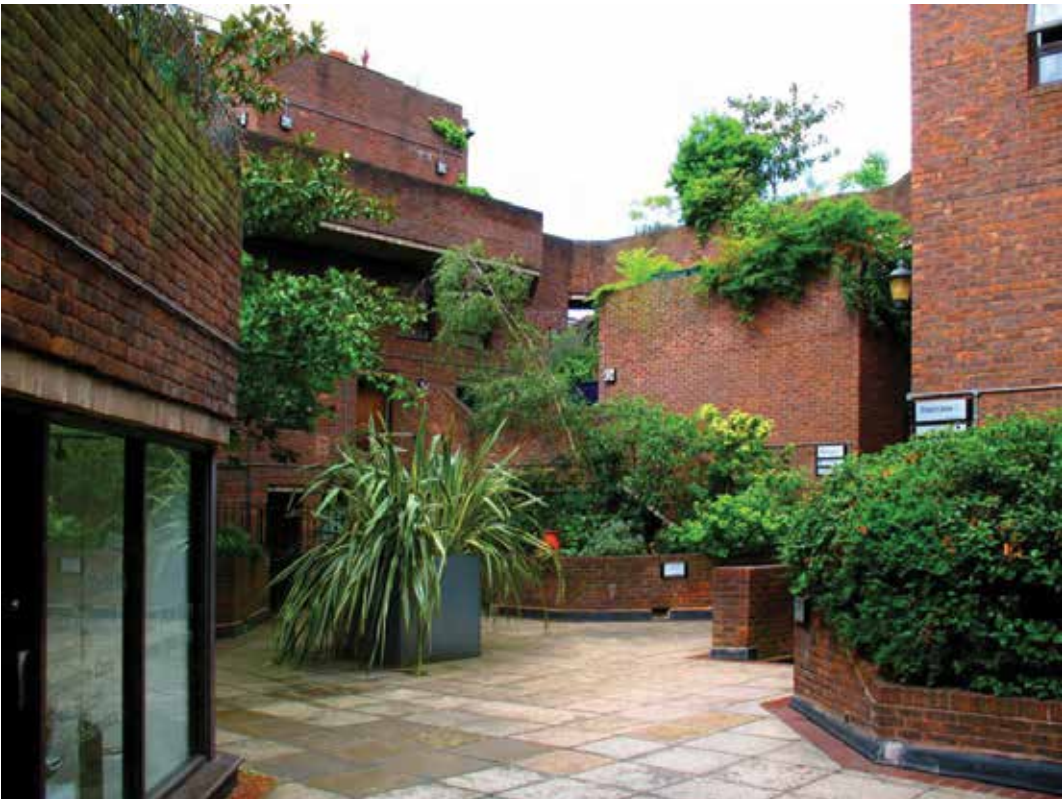
The structure of Odham's walk is based on a concrete frame with hollowcore floor slabs. This system is then covered in a multi-colored stock brick to seamlessly fit the complex into the surrounding Covent Garden neighborhood. Looking closely, however, much of the concrete structure is still visible. The roof insulation is provided by an "inverted roof." The dwellings are heated by individual and centralized gas-fired boilers with central metering.
