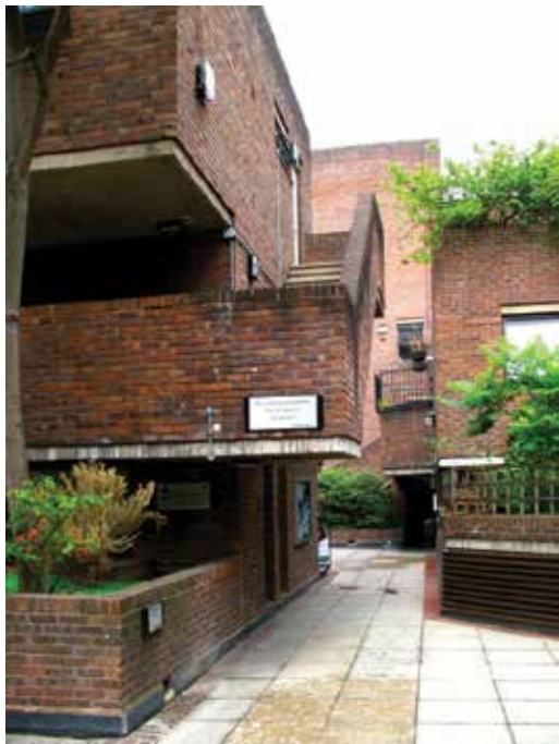
The structure of Odham's walk is based on a concrete frame with hollowcore floor slabs. This system is then covered in a multi-colored stock brick to seamlessly fit the complex into the surrounding Covent Garden neighborhood. Looking closely, however, much of the concrete structure is still visible. The roof insulation is provided by an "inverted roof." The dwellings are heated by individual and centralized gas-fired boilers with central metering.
