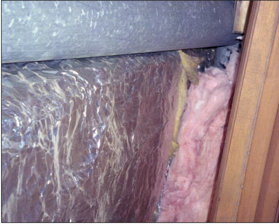
Insulation has been stuffed into the gap in framing between HVAC ductwork and the ceiling framing
