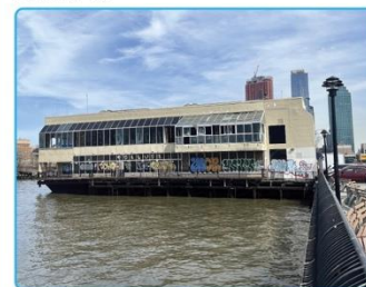
15/ Remove the Dilapidated 'Water's Edge' Barge at 44th Drive
