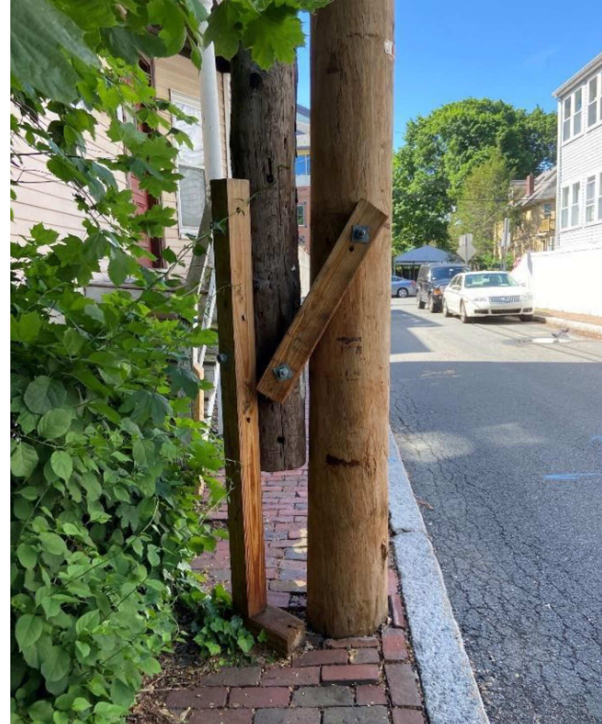
sistering telephone poles
