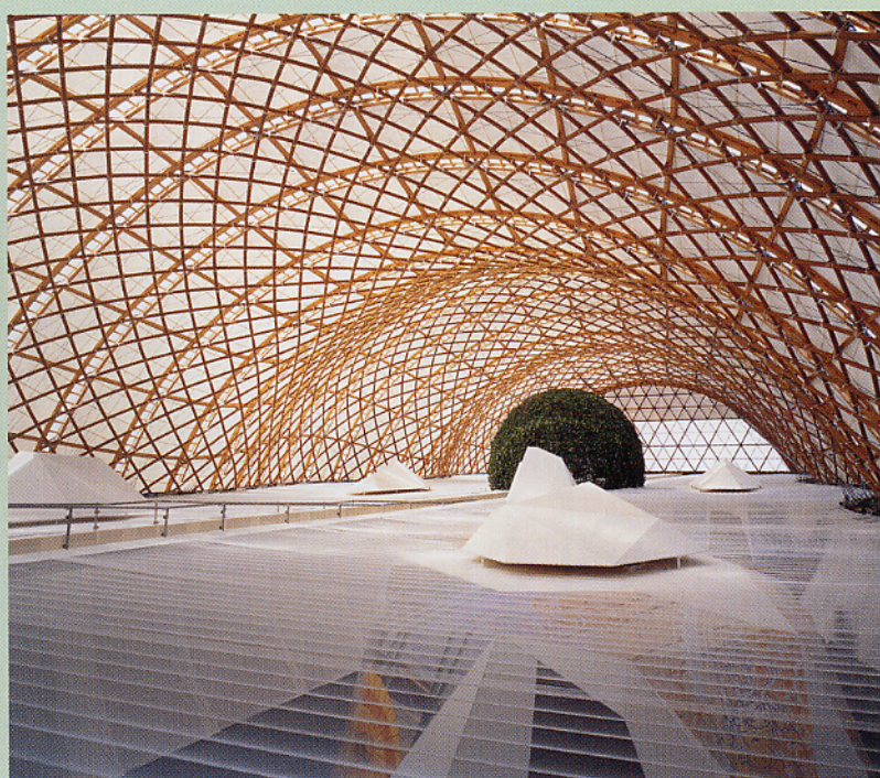
Japan Pavilion, Expo 2000 , upper level of main exhibition space, with roof constructed of paper tubes, fabric tape, wood arches, and paper membrane reinforced with fiberglass and laminated with P.V.C., 2000. Hannover, Germany.
