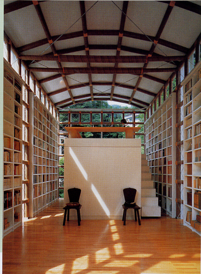
Library of a Poet , permanent building constructed of paper tubes, wood joints, prefabricated bookshelves, steel rods, and wood flooring, 1991. Zushi, Kanagawa, Japan.
