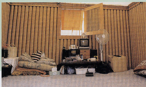
Paper Log House , living space in a completed log house, temporary relief shelter constructed of paper tubes, sponge tape, plywood, beer crates filled with sandbags, and a P.V.C. tent membrane, 1995. Nagata, Kobe, Japan.
