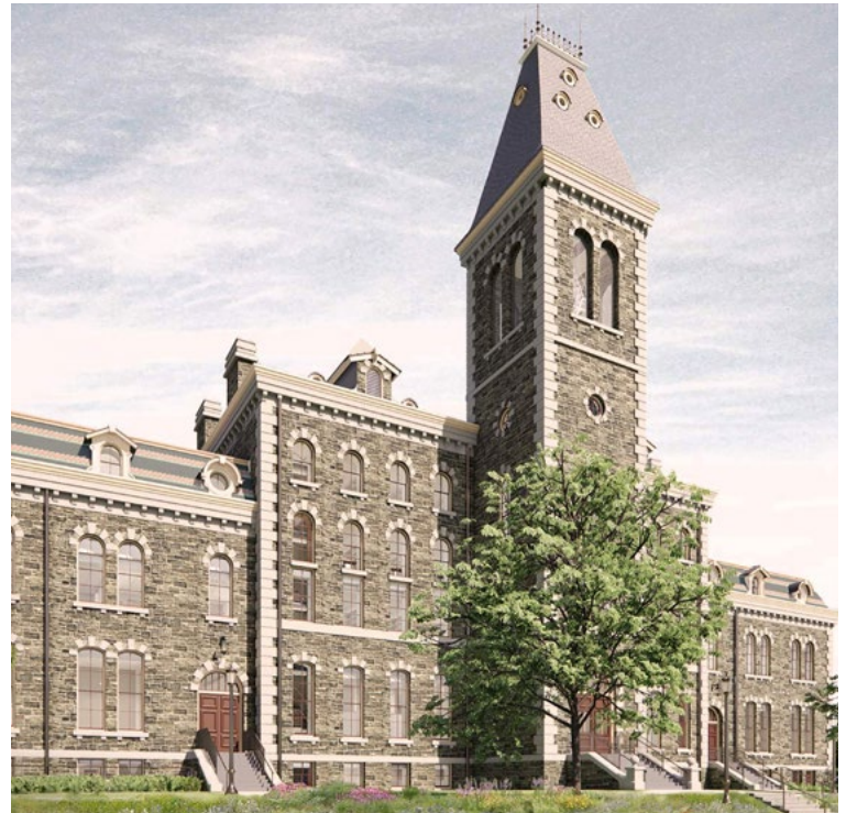
McGraw Hall Adaptive Reuse – Ithaca, NY Professional, 2024, Beyer Blinder Belle—Conversion of a key building on the Cornell Quad into lecture, classroom, & offices for the anthropology department, as well as a change in access and surrounding landscape.
