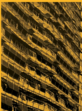
Marcelo and Mauricio Roberto Apartment building in Rio De Janeiro 1956
