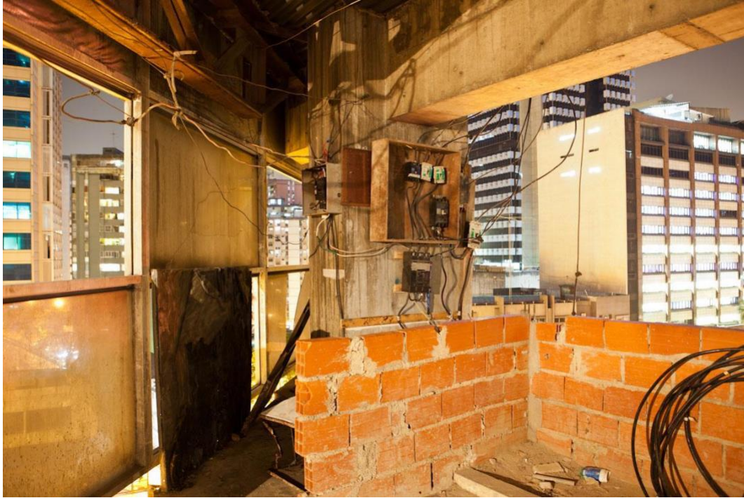
Figure 2. Photograph of Resident's Self-Constructed Electrical Infrastructure within the Tower connecting to the State Electrical Grid. Iwan Baan, Urban Think Tank (2012).
