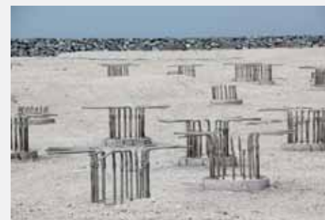
Foundations laid for the Guggenheim Abu Dhabi. © Guy Mannes-Abbott
