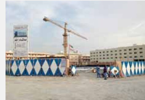
Labour camp construction boom. ©Guy Mannes-Abbott
