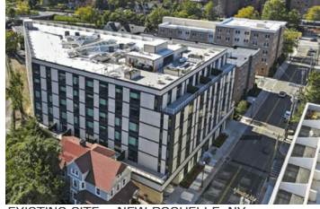
EXISTING SITE - NEW ROCHELLE, NY
