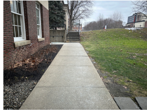
View leading to ADA ramp
