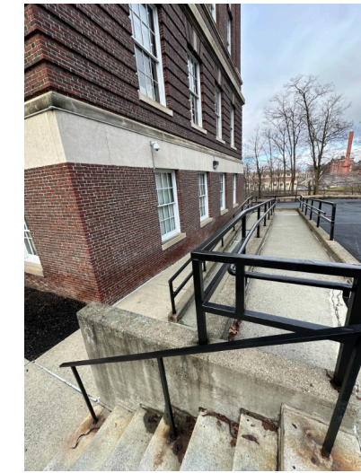
View of ADA ramp
