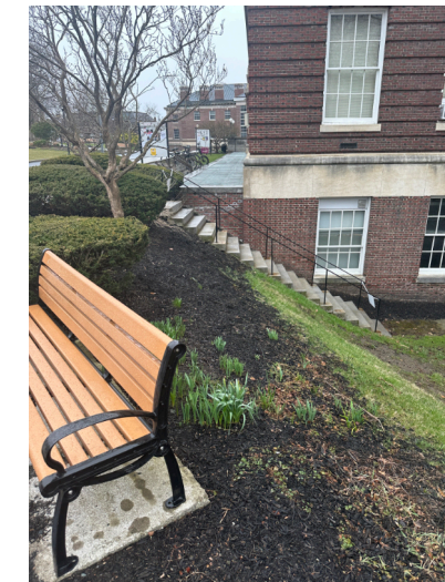
Existing Bench and stairs
