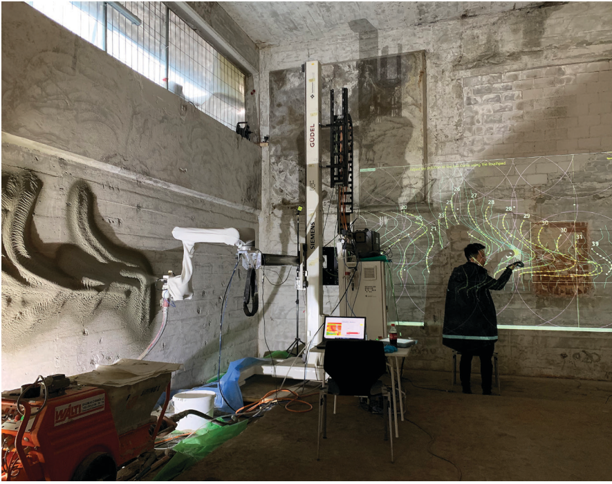
Figure 1. IRoP, interactive robotic plastering system.
