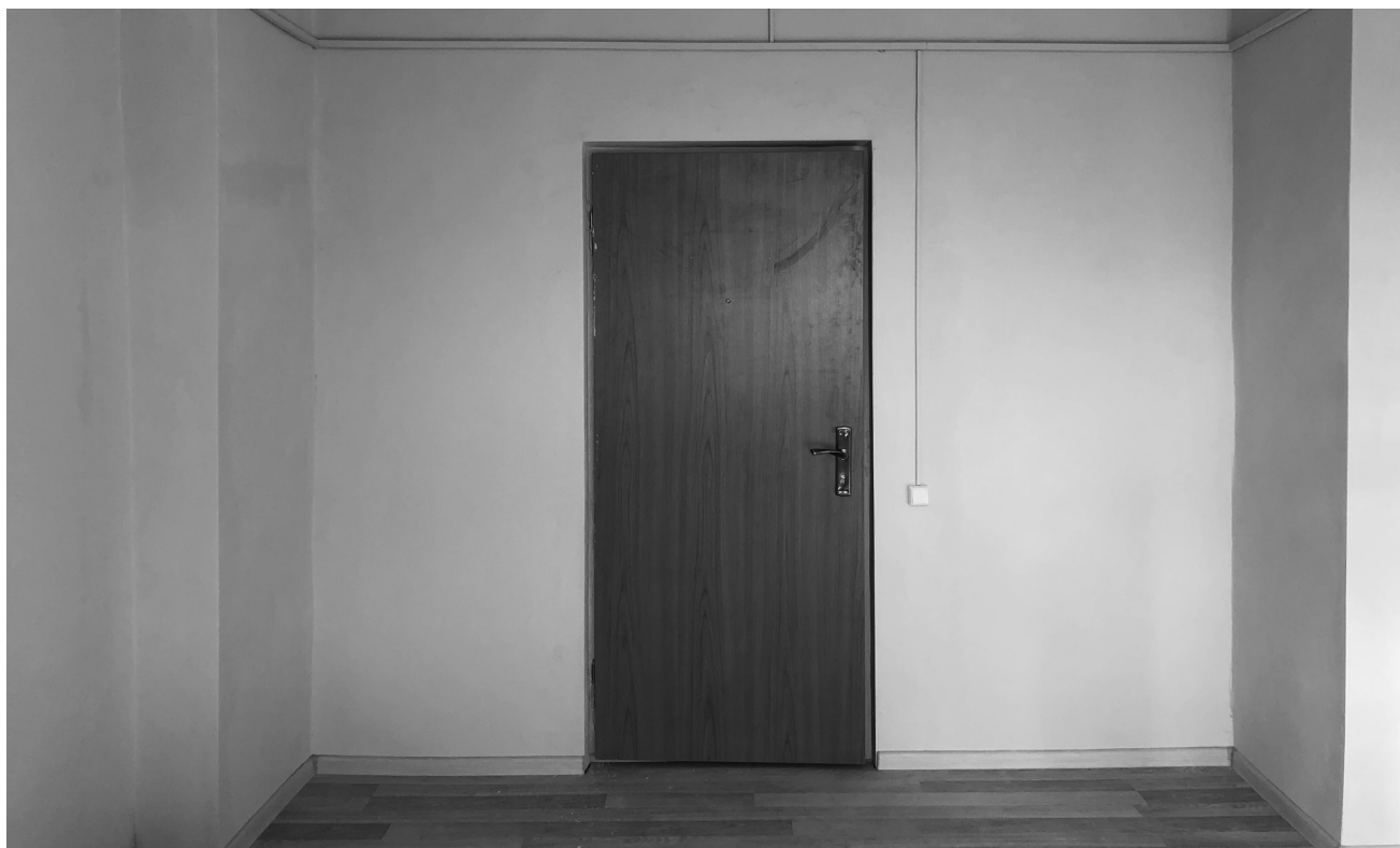
Installed door donated by Re-WIN for CO-HATY shelter in Kamyanets-Podilsky, March 2024.
