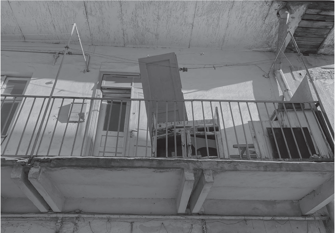
Balcony on the rear facade of the building. Photo: Anna Pashynska, 2024
