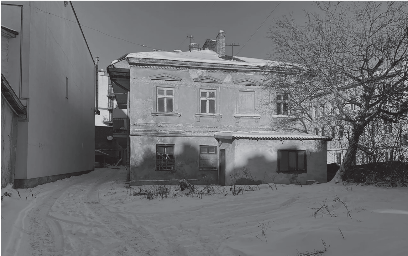
Vacant building, view from Chimichna street. Photo: Anna Pashynska, 2024
