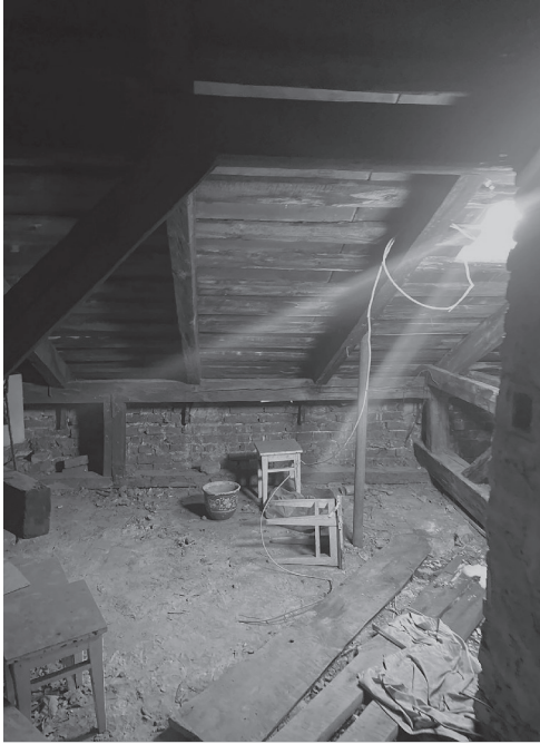
Attic in the vacant building. Photo: Anastasiya Ponomaryova, 2024
