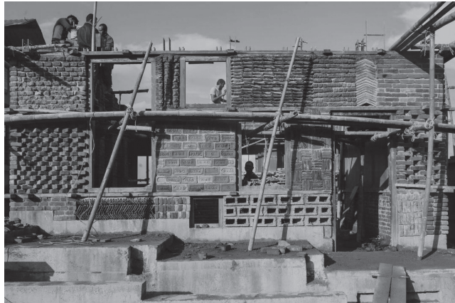
Brickhouse, Nepal project by Superstructure gUC. Photo: Superstructure gUC
