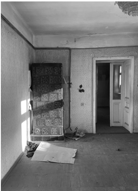
Vacant Building in Lviv. View from the one of the living room. Photo: Anastasiya Ponomaryova, 2024
