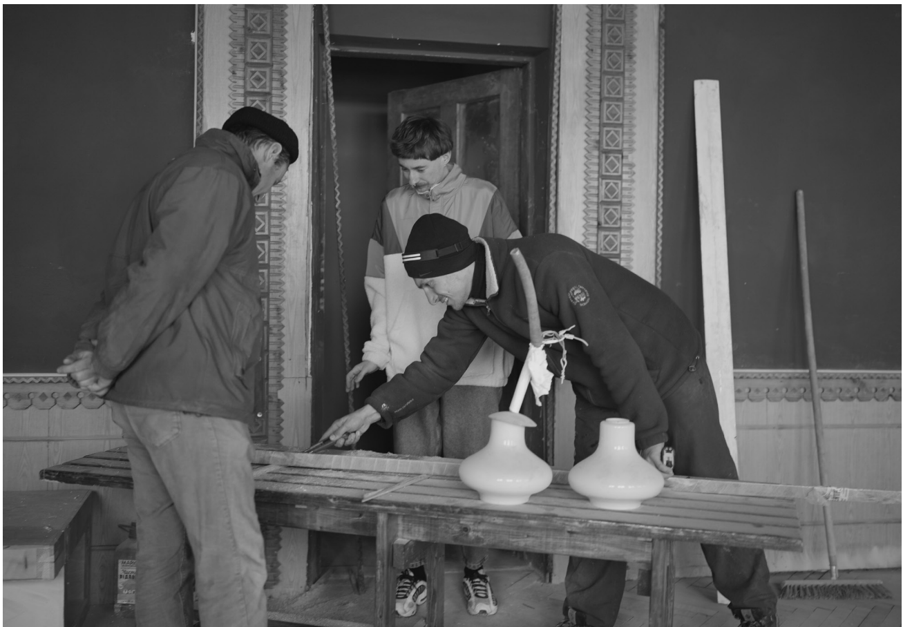
CO-HATY shelter. Construction process, July 2022. Photo: Oleksandr Demianiv ©METALAB
