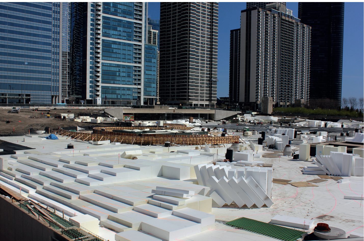
FIGURE 4.2.1 Installation of Geofoam at Maggie Daley Park
