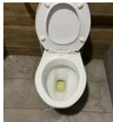
Unflushed toilet, wet floors
