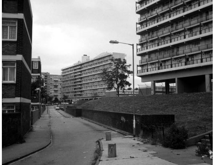
C. G. Weald and Colin St. John Wilson, for the London County Council Architects Department, Bentham Road estate, Vaine House (center), Granard House (right), 1959.
