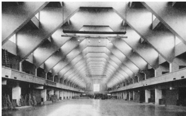
The triangular truss system of the Broadcasting House, Berlin
