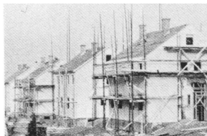
Scaffolding erected for painting
