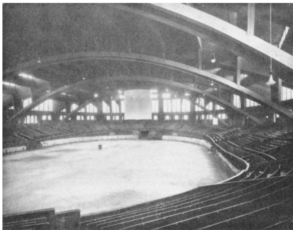
The rafter and bracing system of the Westphalia Hall
