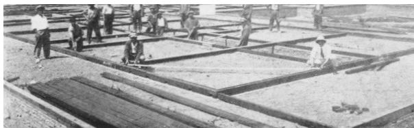
Erection of the ground floor wall panels and assembly of the ceiling beams
