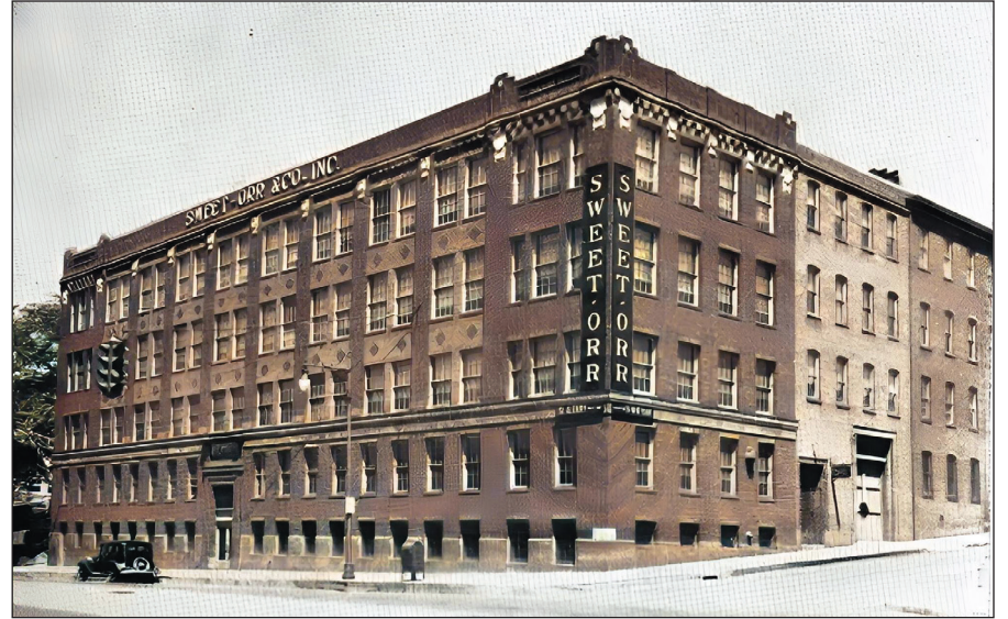
The solid Sweet-Orr building on Broadway demolished after the company moved south.
